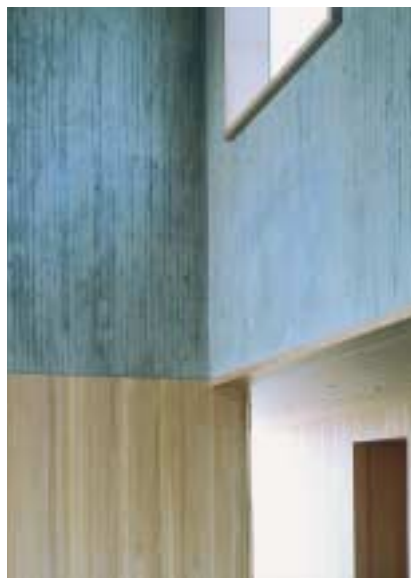
2. Timber cladding with boardmarking above.
