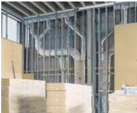
7. Air-conditioning ductwork being concealed behind thick walls.
