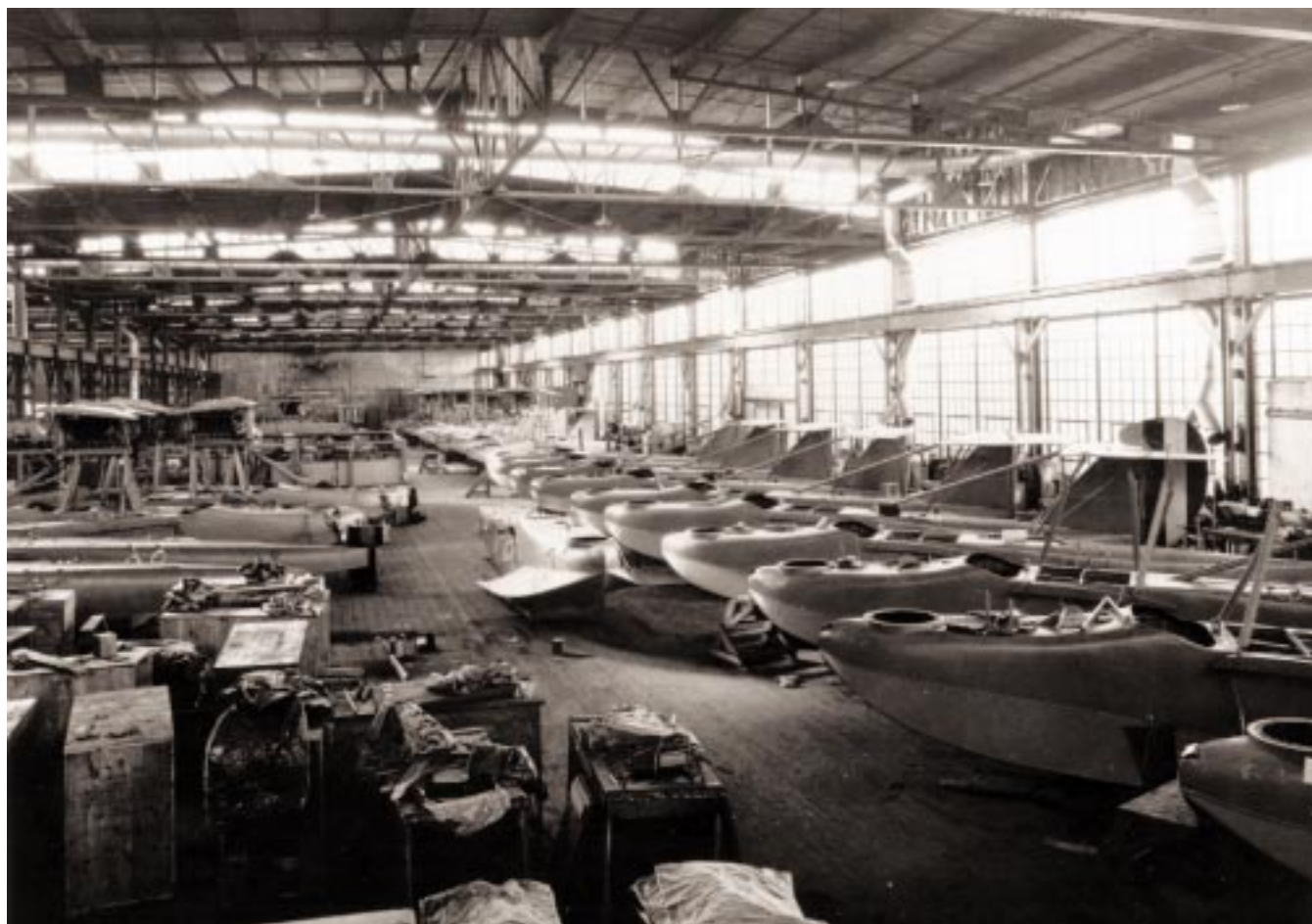
HS-1s under construction.
