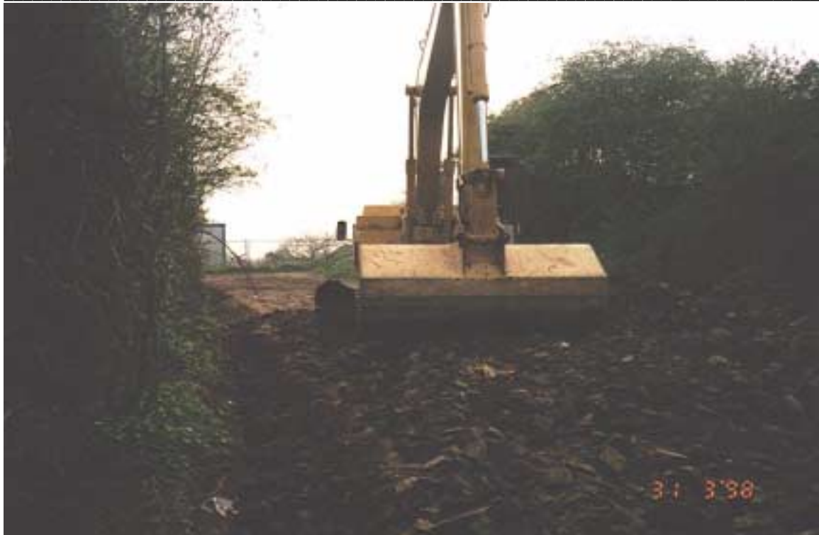
Figure 4.3: Placement of stone rejects to stabilise path
