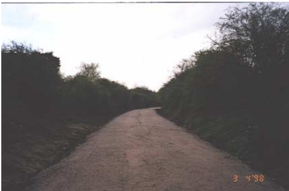
Fig 4.4: Final asphalt surface in place
