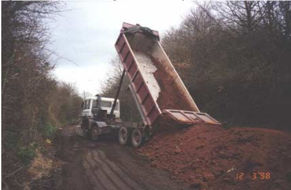
Fig 4.1: Placement of drill cuttings on disused railway line
