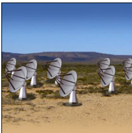
An artist's impression of the dishes of the Karoo Array Telescope on site near Carnarvon in the Northern Cape. Each of the 20 dishes will be 15 m in diameter and about 19 m high. Photograph: Xilostudios
