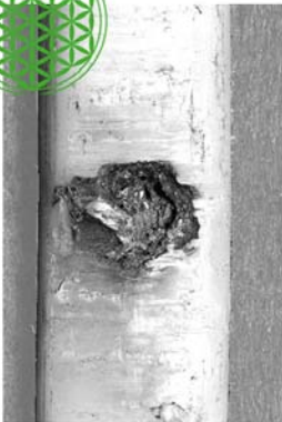
Cable showing shunt fault damage. 'Scrapes' from lateral movement on the seabed and oxidisation resulting from power short are clearly visible.
