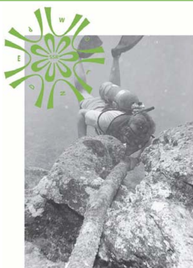
On-site fault inspection by a diver
