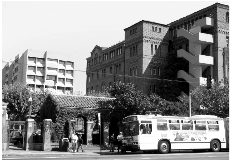
Fig. 3-9 Bus Stop at Main Campus Gate
