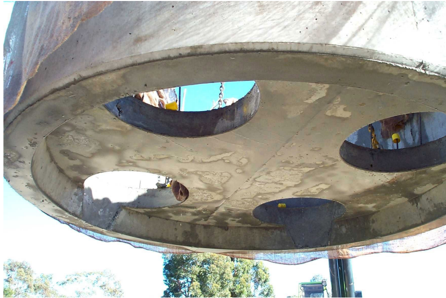
Photo 2 View from underside pilecap shell (courtesy John Holland P/L)
