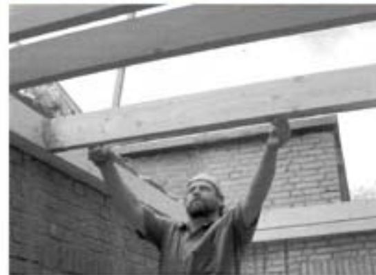
16. Second foundation stone and extension construction (source: Archive Mobarak Mosque)
