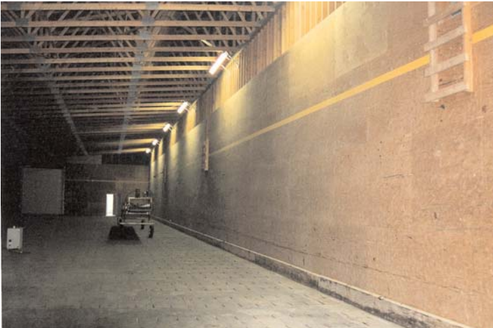
Figure 51: Forced-air storage facilities. Produce is piled up to the yellow line. Air from the floor openings is forced to pass through the stored mass. An inspection alley is located on the upper right-hand side with ladders to sample produce during storage.
