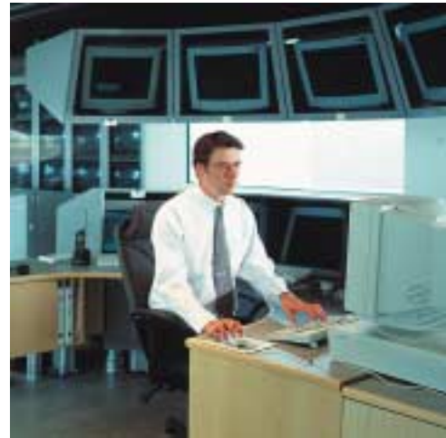
All technical systems are controlled and monitored in the control room.
