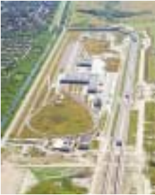
Control and Maintenance Centre, Ørestad.
