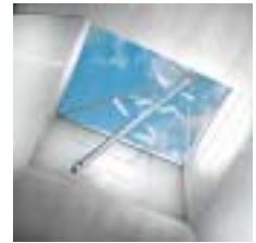
Skylight at tunnel station. Daylight is guided down to the station area, the effect of which is controlled by prisms and other means.
