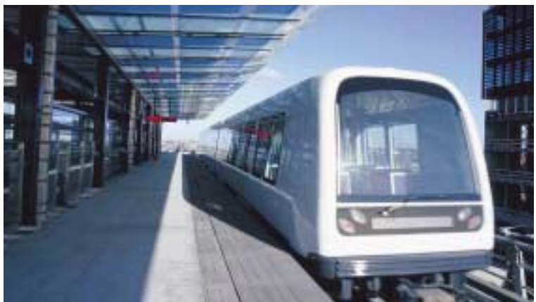
Metro train en route on the elevated track at Ørestad. In all, the elevated track and embankment comprise eleven kilometres of the Metro's total track length.
