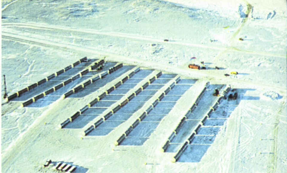
Aerial view of tank farm showing converted fuel tanks being loaded with ice.
