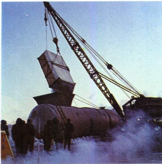
Snow being poured through a specially constructed metal chute into 25,000-gallon tank.
