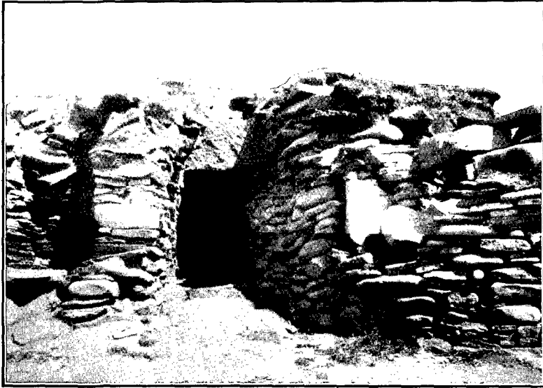
Fig. 5. Opening of Gallery or Passage in the thickness of the Outer Main Wall. From the sea-beach.
