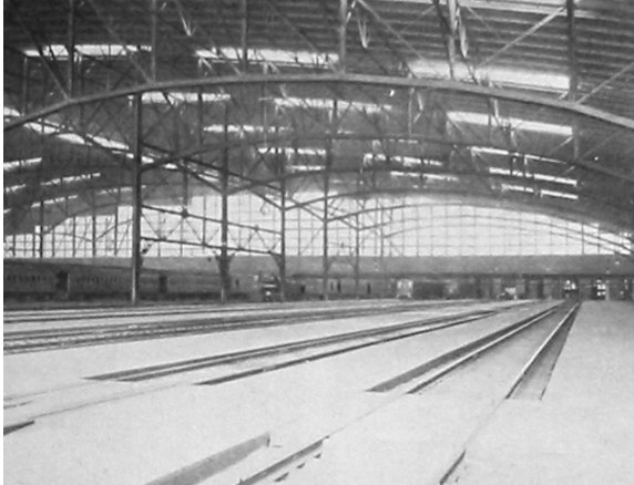
Inside the train shed in South Station (Boston Public Library)
