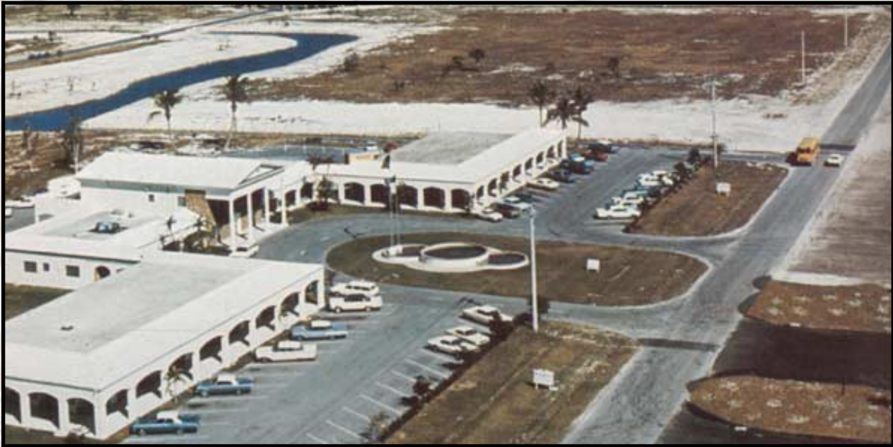
City Hall was originally the Administration Building for the corporate headquarters of Coral Ridge Properties.
