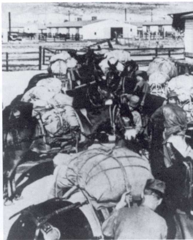
Mule barn area at Camp Carson.
