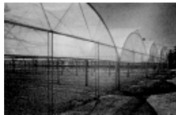
Fig. 12. Tunnel-shaped greenhouses covered with double EVA film.
