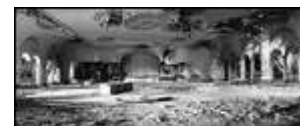
The Grande Ballroom closed in 1972, six years after it opened. This 2003 view of what's left of the interior is from the Fabulous Ruins of Detroit. (LOWELL BOILEAU/Detroit Yes)
