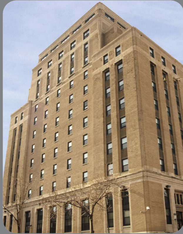
1997 Van Rensselaer Hall, student residence (renovated) Architect: Bower Lewis Thrower
