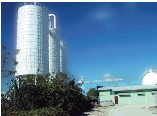
Silos storing cement on Thilafushi Island.
