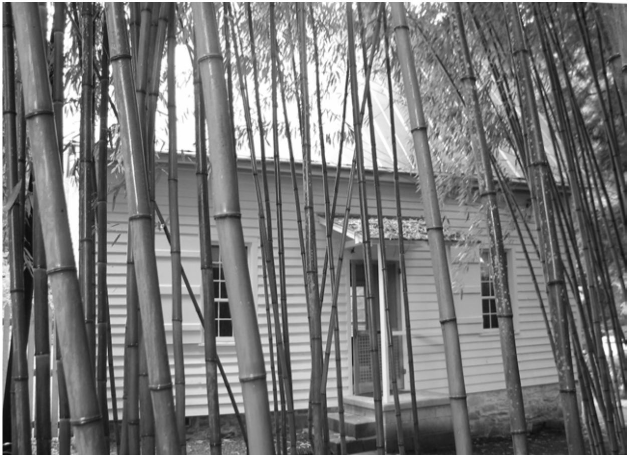
FIGURE 48. View to southwest of front of Swedish House. (T. Jones, NPS, 2004)
