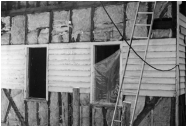
FIGURE 44. View of east end of house after installation of insulation. (CARL4008/03/39P)
