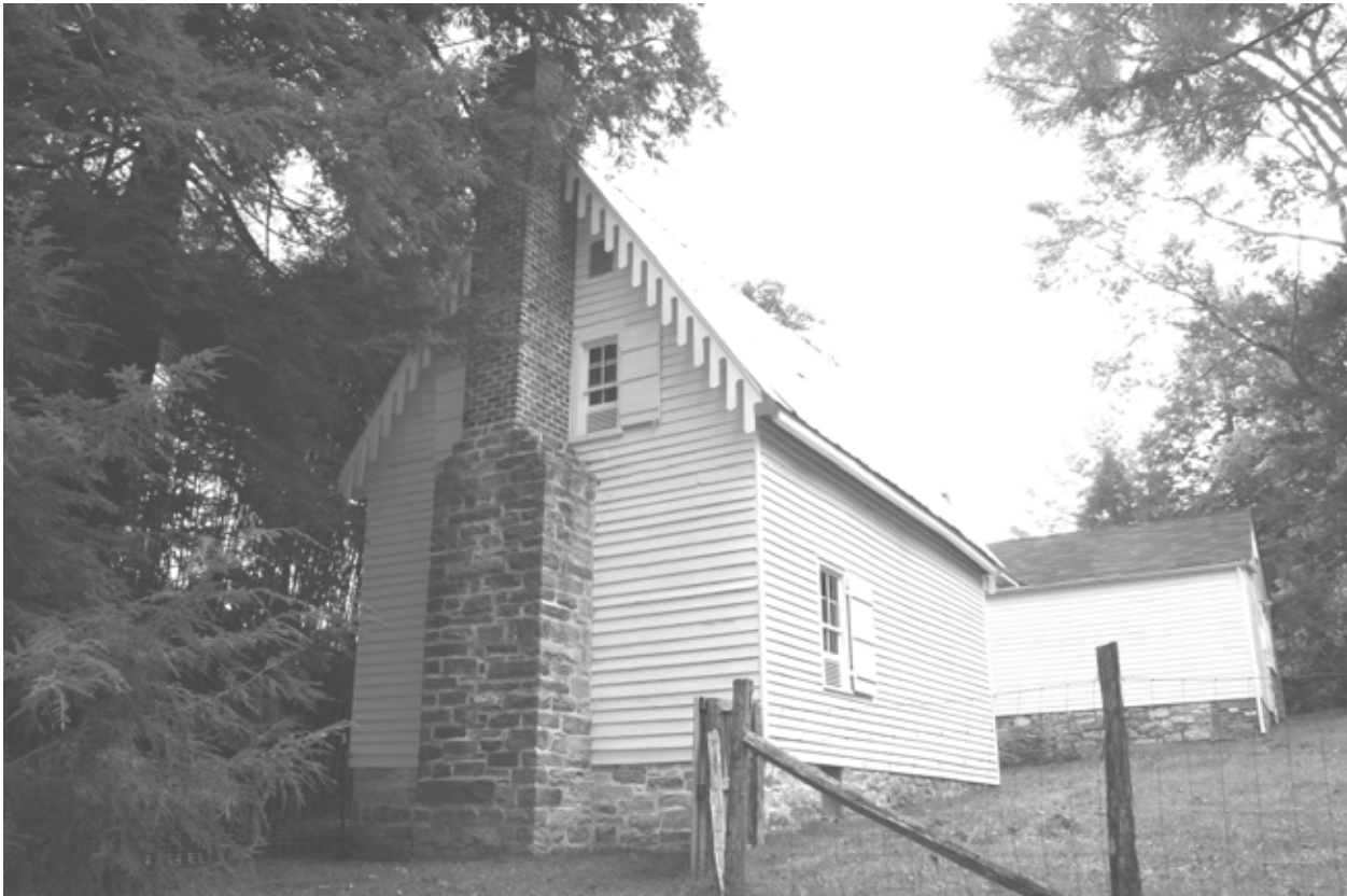
FIGURE 49. View to northeast of rear and west end. (T. Jones, NPS, 2004)
