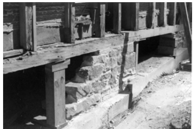
FIGURE 36. View of south foundation during repairs, 1977. (CARL4008/03/25P)
