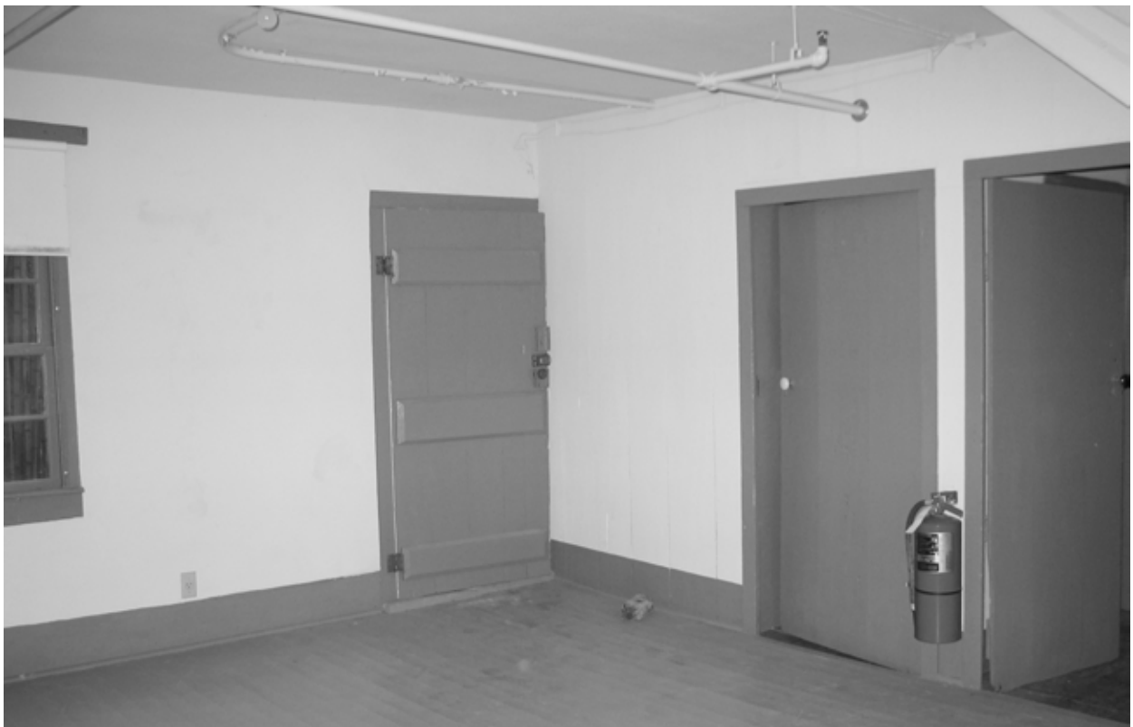
FIGURE 57. View northeast in Room 100. (T. Jones, NPS, 2004)
