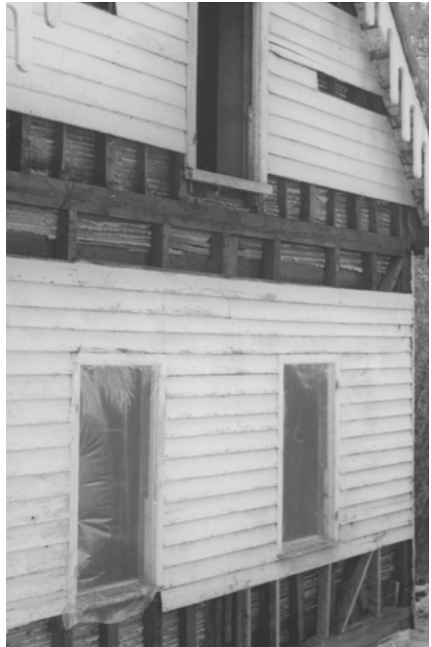
FIGURE 43. View of east end of house, 1977. (CARL4018/02/118P)
