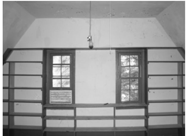
FIGURE 68. View west in Room 201. (T. Jones, NPS, 2004)
