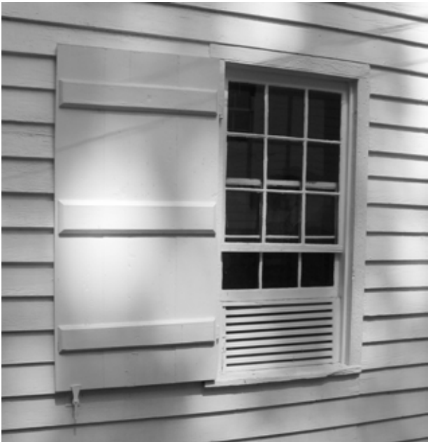
FIGURE 53. View of window on east side of Room 102. (T. Jones, NPS, 2004)
