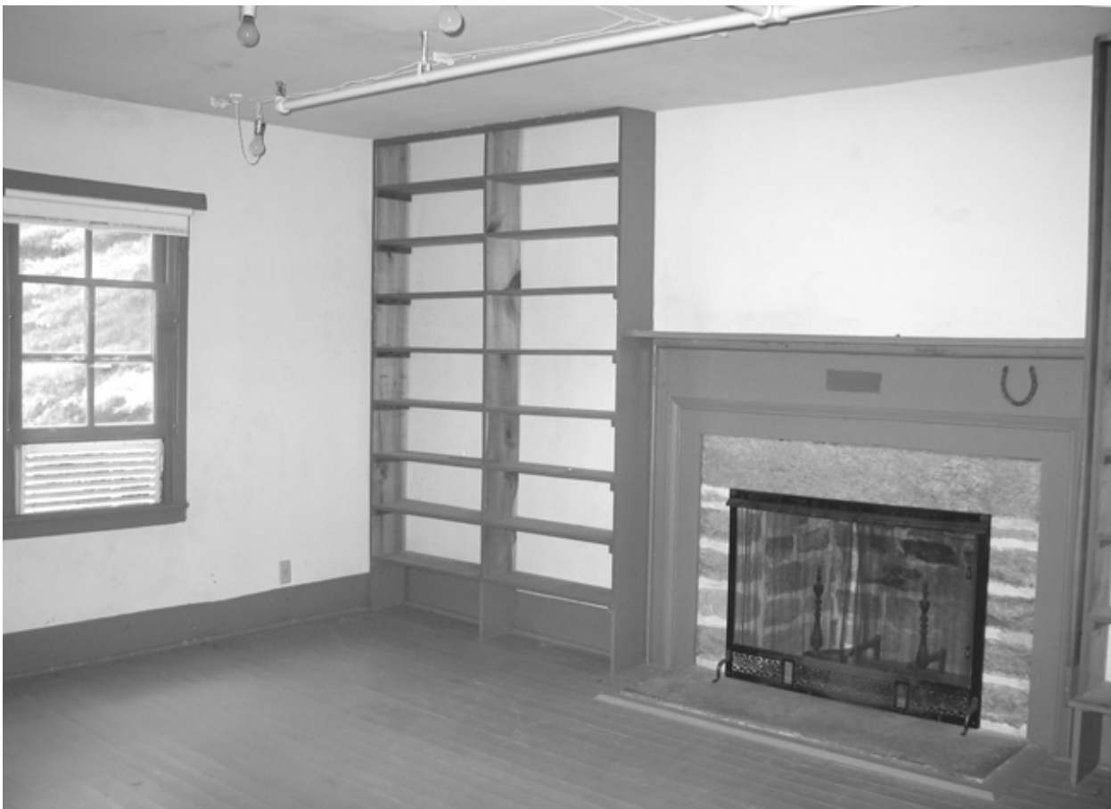
FIGURE 56. View southwest in Room 100. (T. Jones, NPS, 2004)
