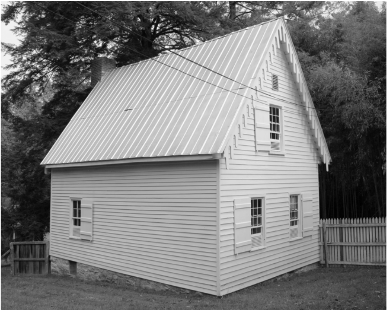
FIGURE 50. View to northwest of rear and east end. (T. Jones, NPS, 2004)
