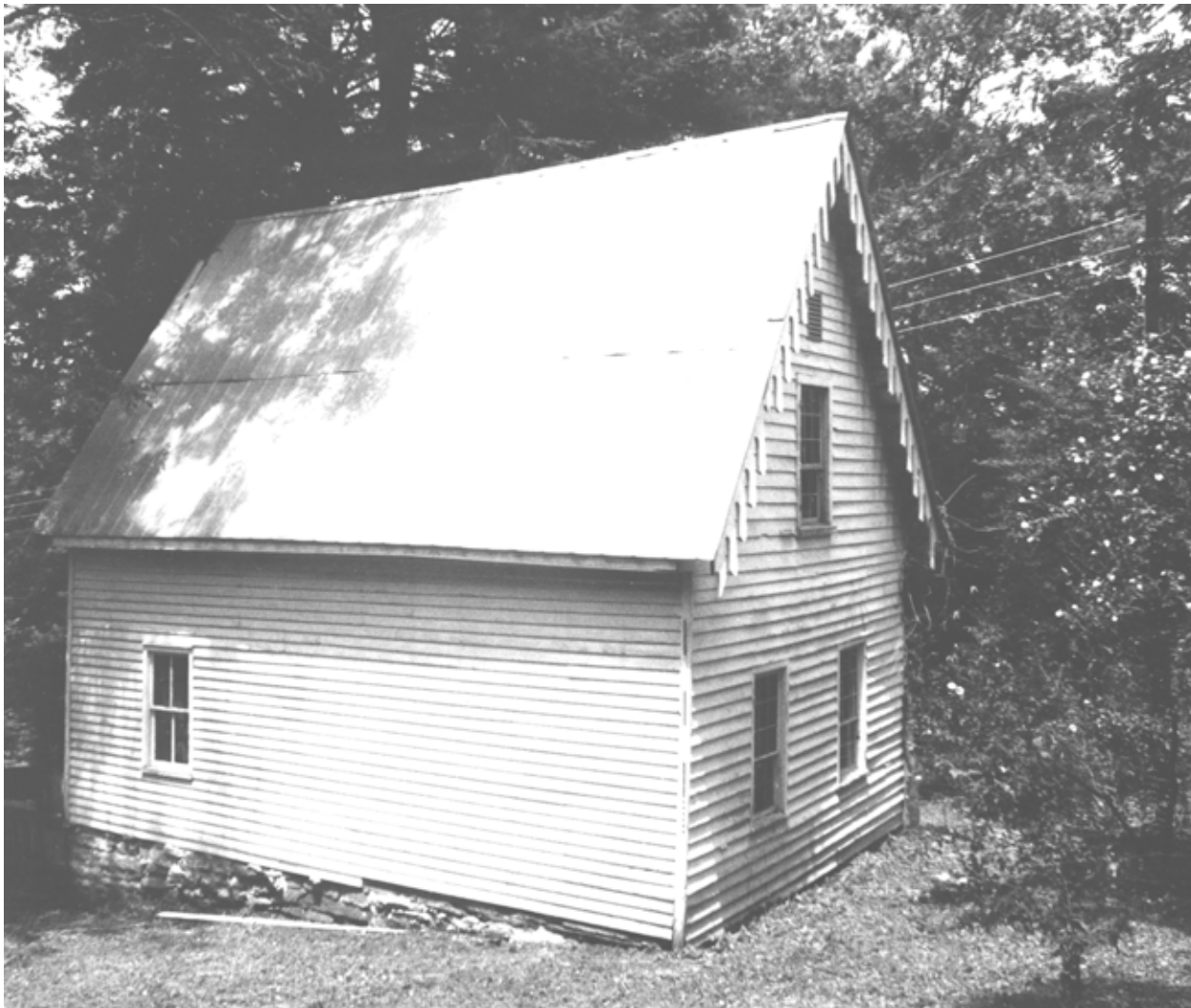
FIGURE 33. View of Swedish House, 1971. (CARL5026/2/3P)
