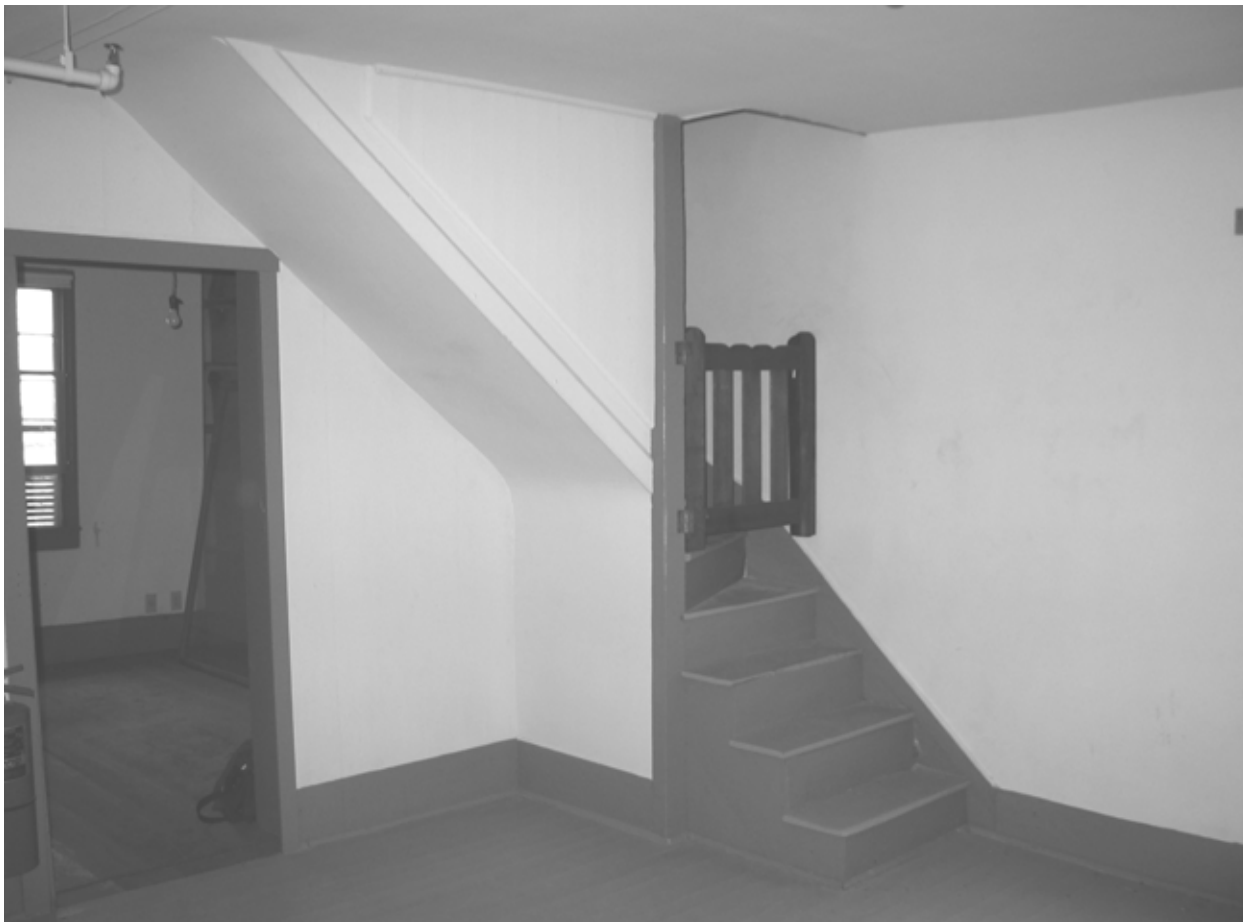
FIGURE 58. View southeast in Room 100. (T. Jones, NPS, 2004)
