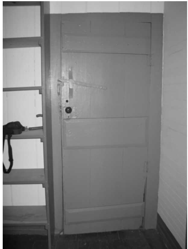
FIGURE 63. View west in Room 102. (T. Jones, NPS, 2004)
