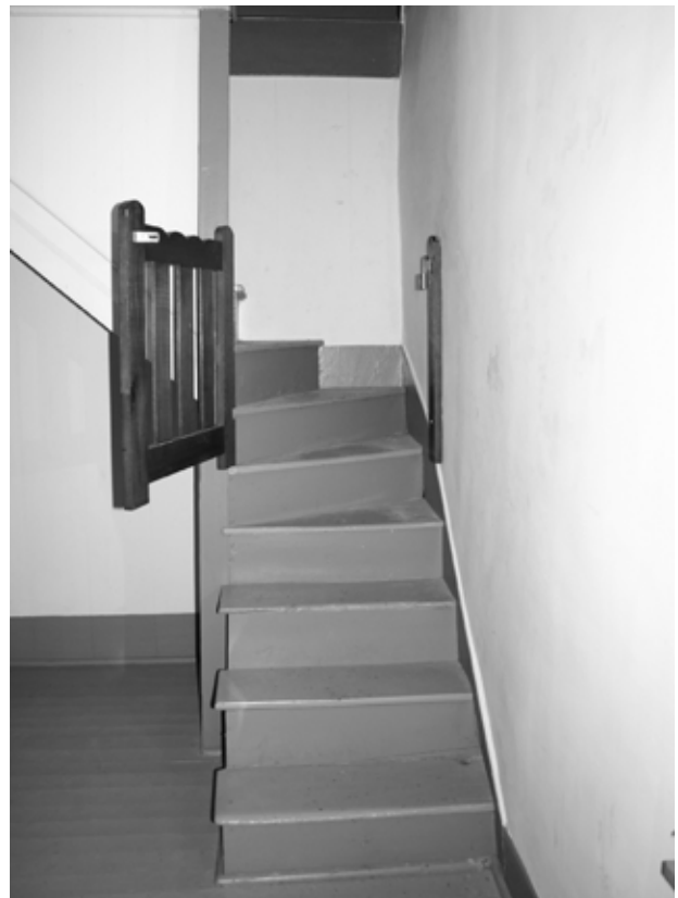
FIGURE 64. View of stairs to second floor. (T. Jones, NPS, 2004)
