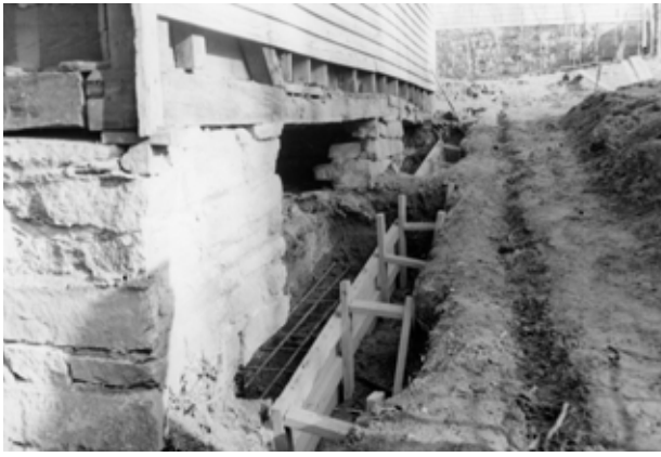
FIGURE 39. View of new footings, 1977. (CARL4008/03/15P)
