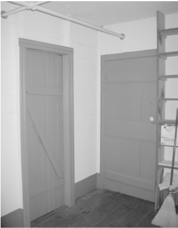
FIGURE 61. View southwest in Room 101. (T. Jones, NPS, 2004)
