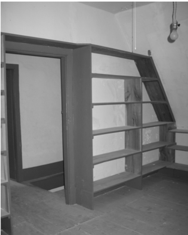
FIGURE 66. View southeast in Room 201. (T. Jones, NPS, 2004)
