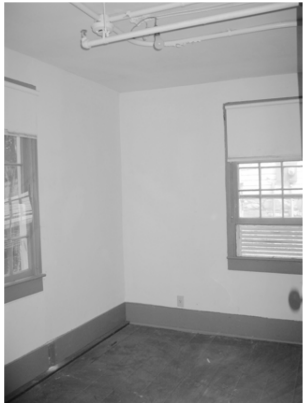
FIGURE 60. View northeast in Room 101. (T. Jones, NPS, 2004)
