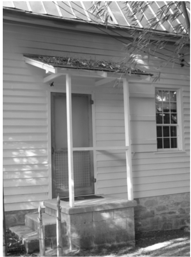
FIGURE 54. View of twentieth-century stoop and shed roof at front door. (T. Jones, NPS, 2004)
