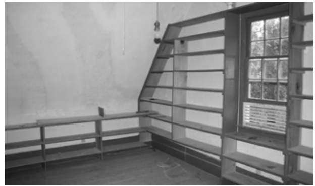
FIGURE 67. View northeast in Room 202. (T. Jones, NPS, 2004)
