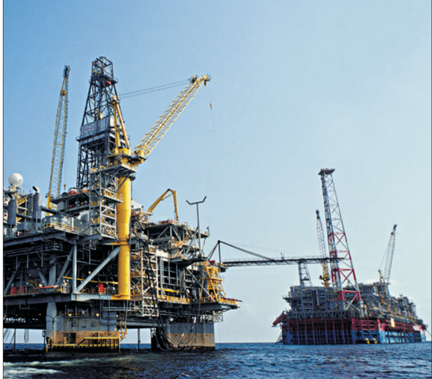
The world-class Kizomba A project includes the world's largest FPSO vessel (2.2 million barrels) that receives production from a 36-slot tension leg platform.
