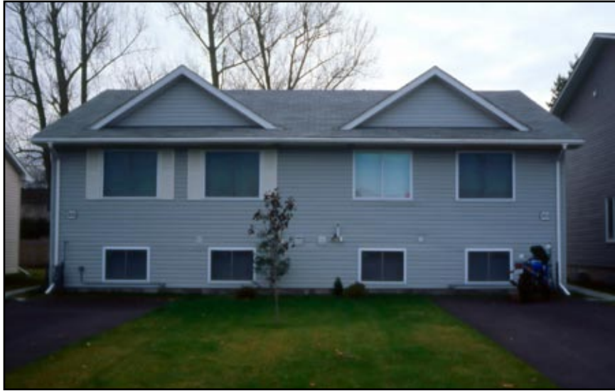
Ottawa: self-sustained affordable housing by Habitat for Humanity.
