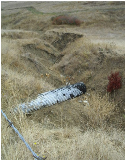
Figure 23. Photographs of a hanging culvert draining Castro Ranch Road, and of the gully that has developed downstream.
