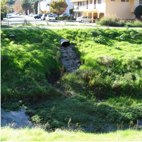
Figure 26. Example of minor channel bank erosion where a culvert draining city streets enters the mainstem channel.
