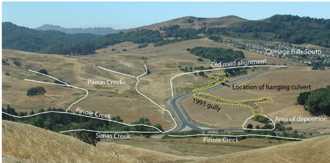
Figure 24. Photograph looking across the valley at Castro Ranch Road and the Pavon Creeks area. Photograph shows the current alignment of the road, past alignment, location of hanging culvert (also shown in Figure 23), gully location (dashed yellow line), and area of sediment deposition.
