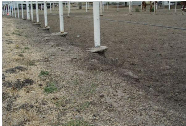
Figure 29. Exposed fence post bases due to surface erosion in a horse pasture.
