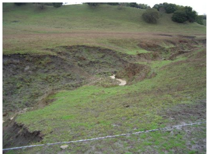
Figure 23. Photographs of a hanging culvert draining Castro Ranch Road, and of the gully that has developed downstream.
