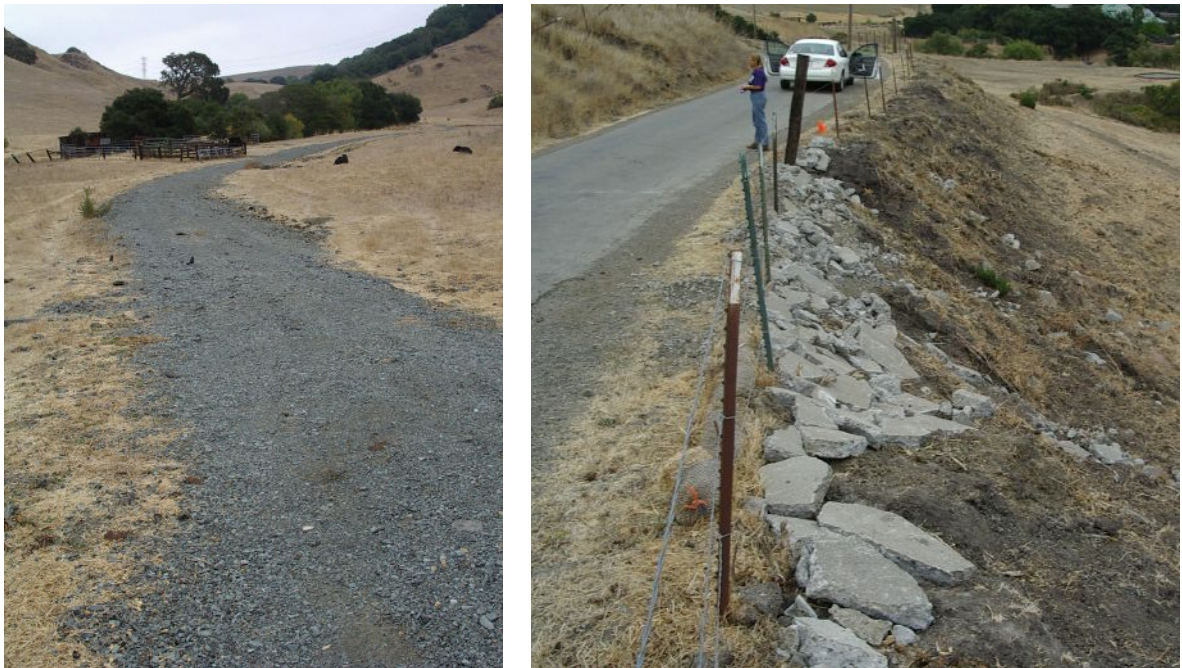
Figure 22. Photos illustrating a well-maintained gravel ranch road, and a poorly maintained paved road.
