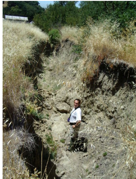
Figure 31. Gully caused by the resultant increase in runoff due to historic removal of topsoil in a sub-basin.
