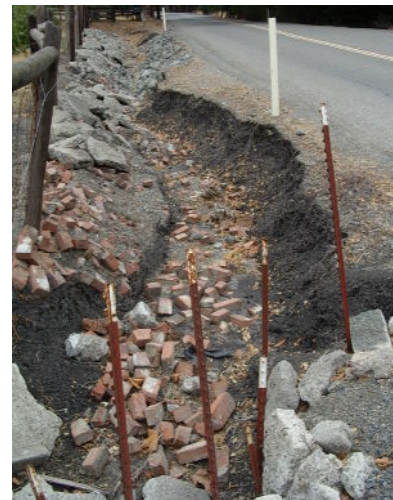
Figure 25. An example of a poorly constructed and maintained inboard ditch that is contributing sediment.
