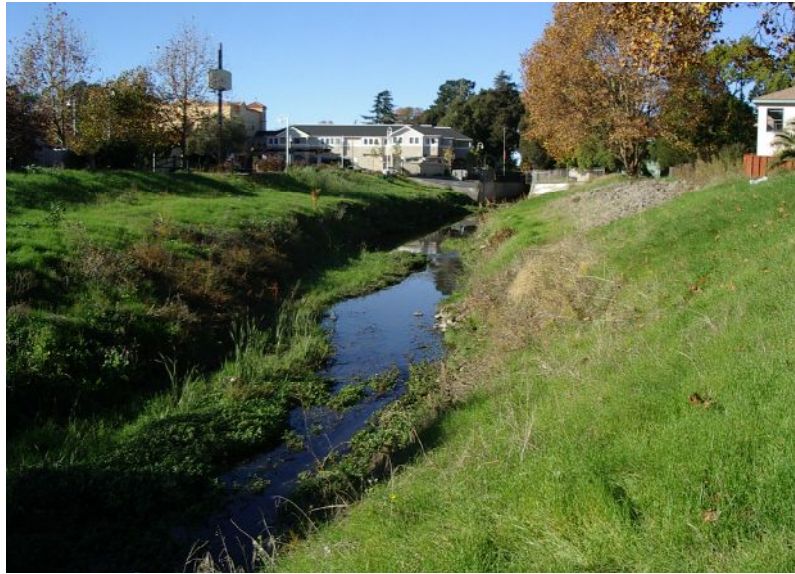
Figure 43. Photograph illustrating typical cross-sectional geometry in the fluvial portion of the flood control channel reach.
