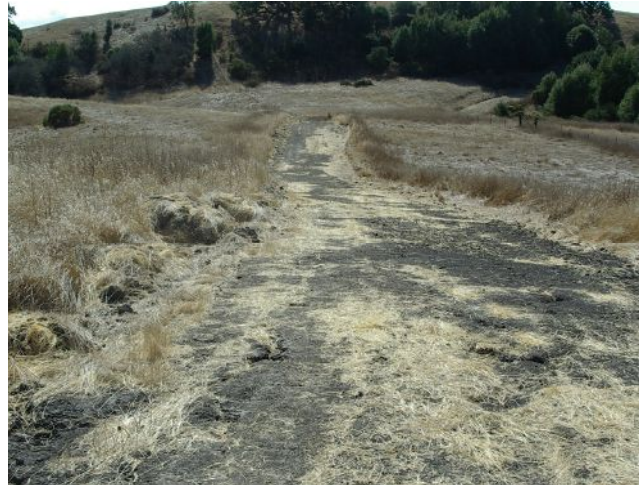
Figure 27. Example of a well-maintained fire trail that is not contributing a significant amount of sediment.
