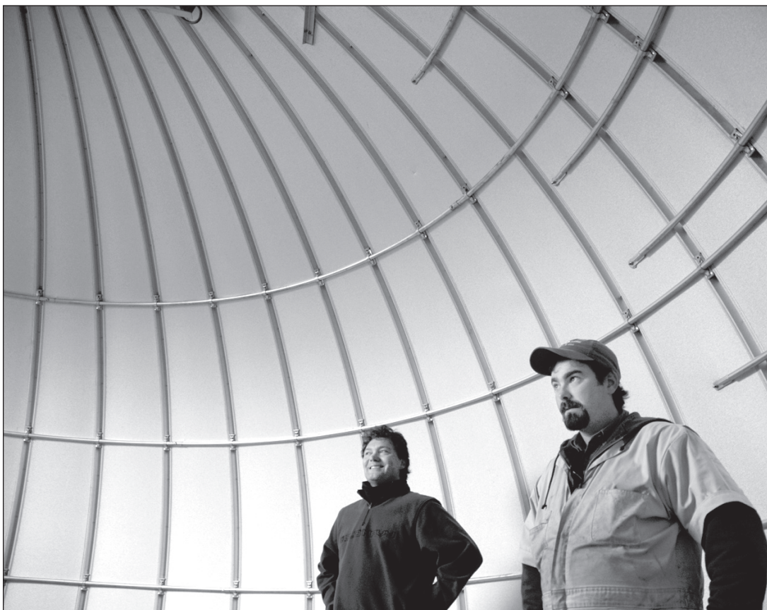
Above: Brian Super of Ash Manufacturing Company holding the galvanized steel dome steady against the wind Friday as it moved into place atop Custer Institute's observatory in Southold. Left: Mr. Super (right) and Kurt Massey inspecting the inside of the new dome after the 22-foot structure was settled on top of the observatory.
