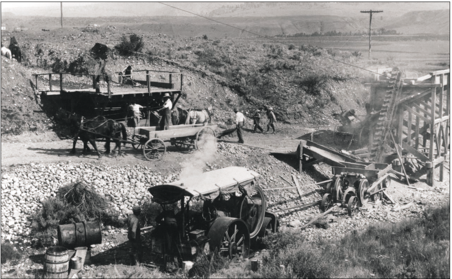
Figure 4. Gravel mining and crushing rock for Omak Streets, 1913. Crushing cobbles and small boulders in 1913 was a labor-intensive process compared to present-day gravel mining operations. Rocks too large to be used as aggregate were crushed to a usable fragment size. The process illustrated in the photo began with screening gravel, including large boulders, through a grizzly (upper left of photo), which was made of wood with cracks narrow enough to keep boulders too large to be crushed from going to the crusher. Some of the boulders are piled up behind the road roller (bottom center of photo). The fraction that passed through the grizzly was then transferred by wheelbarrow (center of photo) to a jaw crusher (center right of photo). The road roller was used to drive the crusher and to power a bucket-line conveyor. The conveyor transferred the newly crushed material to a storage bin. Horse-drawn wagons then transferred the aggregate to the streets of Omak. An empty wagon is crossing in front of the grizzly in the center of the photo and another wagon is loading from the storage bin. Photo courtesy of Cheney Cowles Museum, Spokane, Wash.
