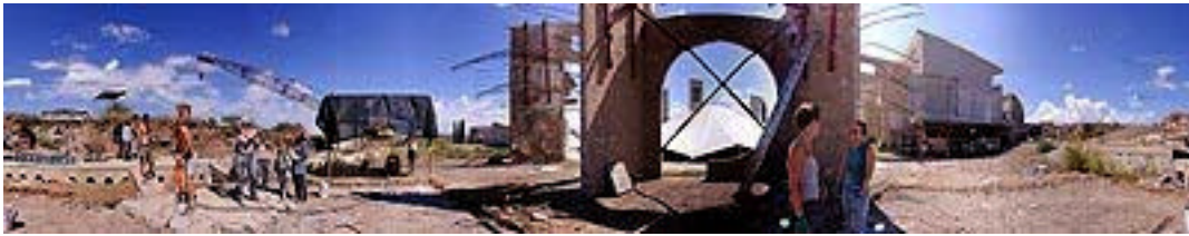
Arcosanti: East Crescent under construction, 1999
