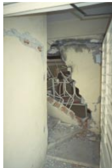
Fig. 18 This building seems nearly undamaged from the outside (left), while the partition walls inside are completely destroyed (damage grade 3)
