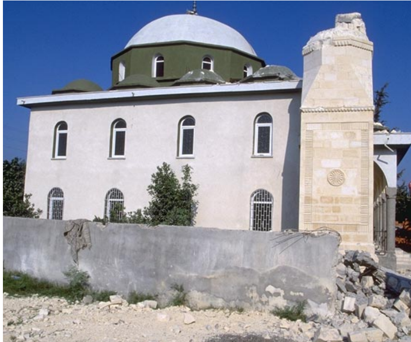
Fig. 29 Mosque with collapsed minaret in Ceyhan
