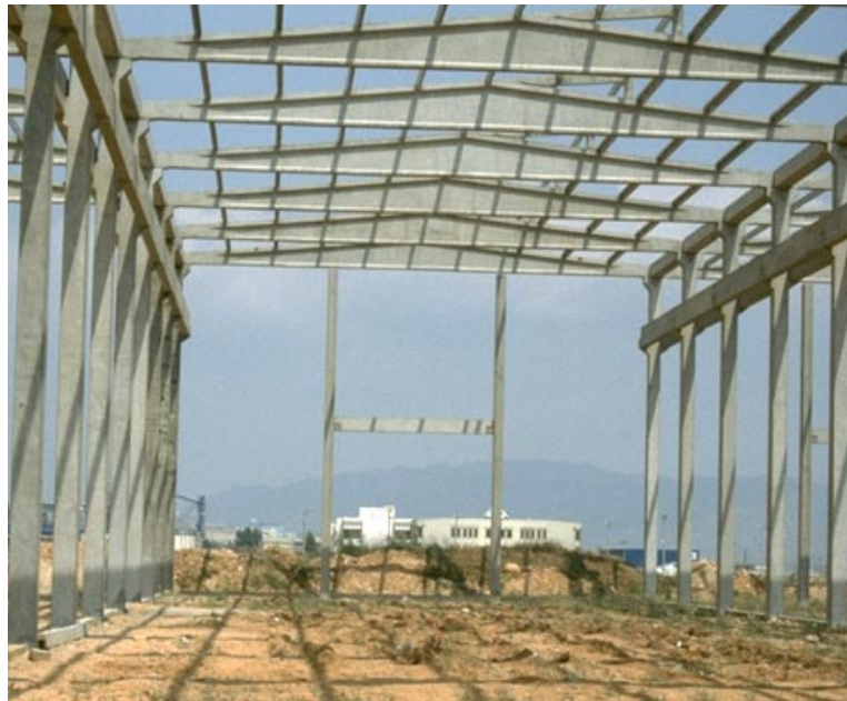
Fig. 24 Typical industrial buildings under construction showing precast reinforced concrete pin-connected frames
