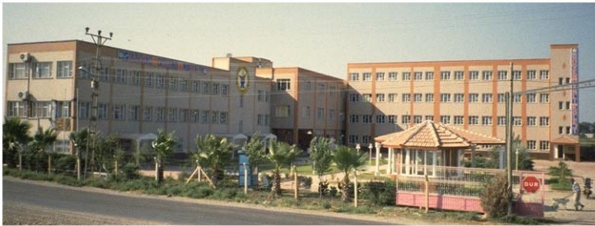
Fig. 22 School buildings west of Ceyhan with damage of grade 2 to 3
