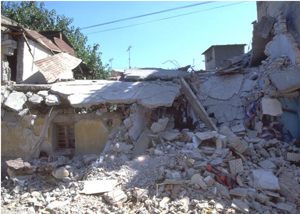
Fig. 31 Collapsed older masonry building in the center of Adana (damage grade 5)
