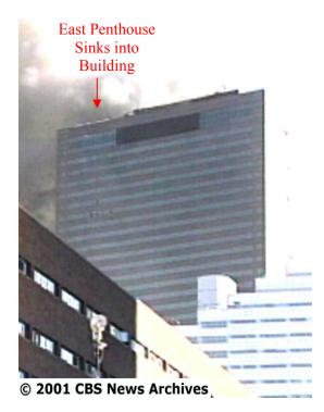
Figure L–26. East penthouse sinks (2.2 s).
