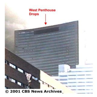
Figure L–27. Center screenwall and west penthouse sink (7.9 s).
