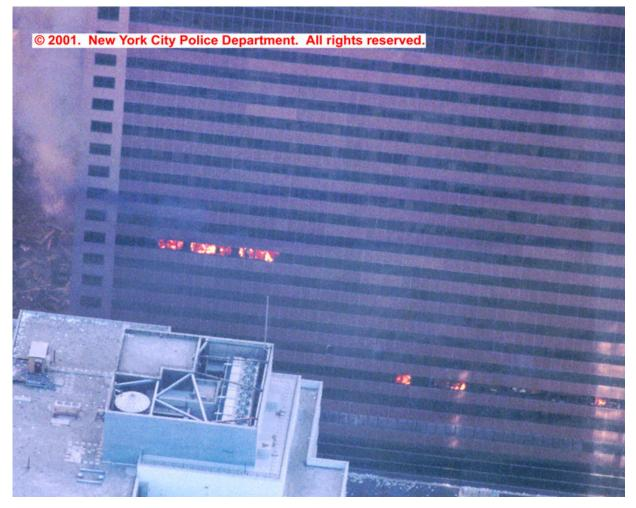
Figure L–24b. Fires on Floors 7 and 12 on the north face.
