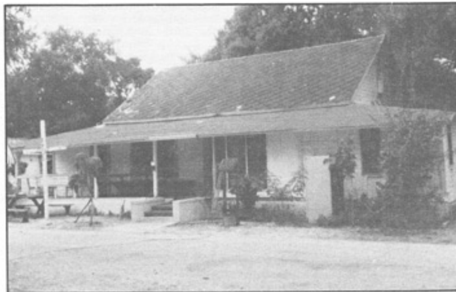
House where Dr. Thomas E. Will lived in the late 1920s, located on Southwest 6th Avenue between Southwest 2nd Street and Southwest 3rd Street, Fort Lauderdale.
