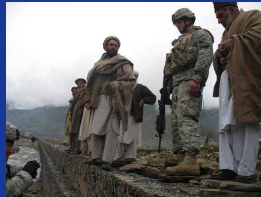
Alishang District Administrator Mohammad Qasim, right, Air Force Lt. Col. Brad Bredenkamp, center, Alishang elder Asadulla Khan, left, and others stand on the newly finished flood protection wall next to Dumlam village in northern Laghman.
