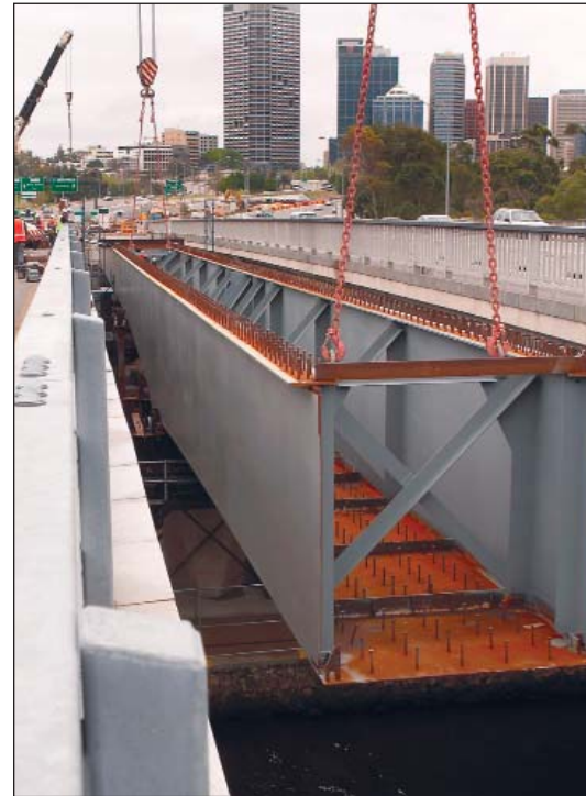
A massive steel girder is lifted into place at the Narrows Bridge
