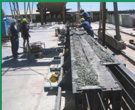
First masts being poured at Delta Concrete
