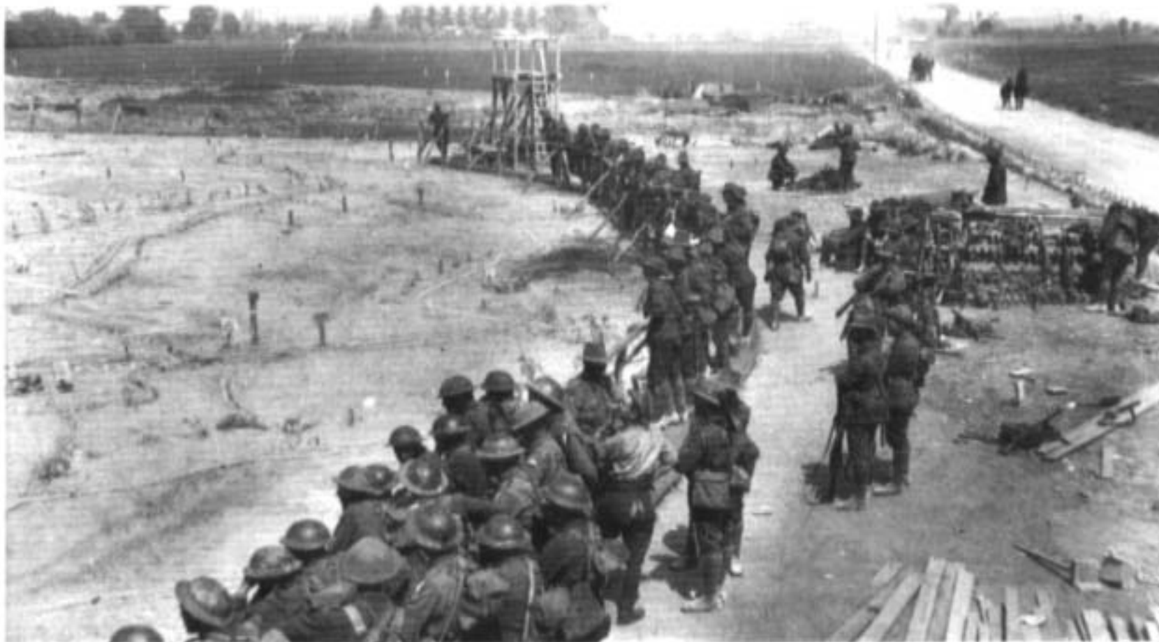
Troops of the Australian 13th Brigade study a map model near Petit Pont, Belgium, on 6 June 1917 in preparation for the next morning's attack on Messines. Construction and updating of the model was the work of engineers and members of the Corps Topographical Section. (AWM F00632)
