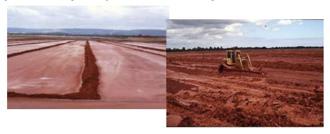
Figure 3 Spreading the slurry, and ploughing using a D6 Swamp Dozer to enhance the drying rate
