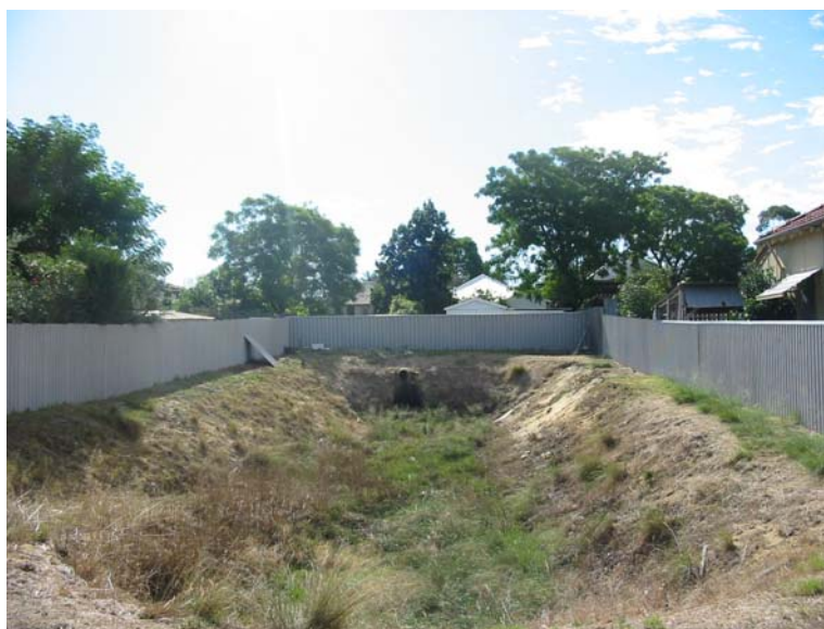
Plate 1. A Sump with little aesthetic value - 39 Esperance Street
