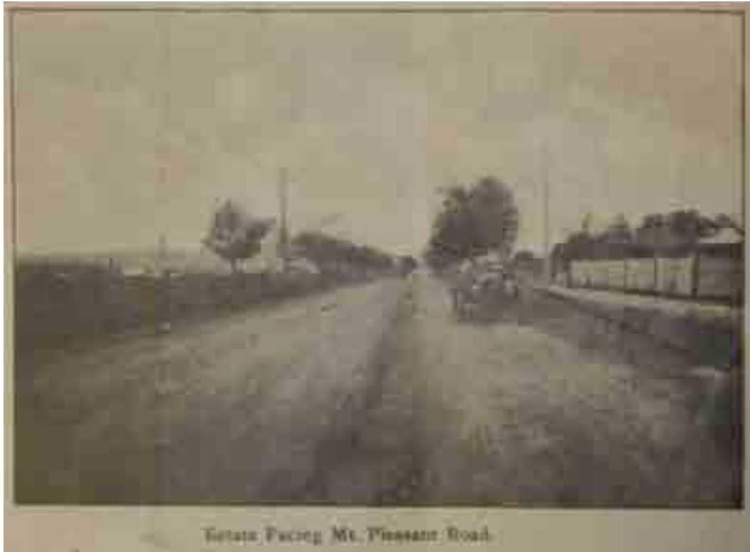
Figure 3.6: Mount Pleasant Road looking east, 1923, with the open paddocks of the Elderslie Estate to the left and properties with front fencing to the right. Also note the roof tops of the dwellings in Seaview Parade and Riverview Terrace in the background. Source: Elderslie Estate subdivision plan, 1 December 1923, Geelong Heritage Centre Maps and Plans Collection, E25.01.
