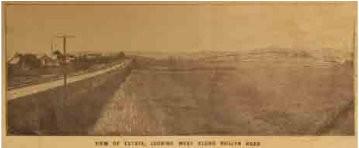
Figure 6.7: View west along Roslyn Road from adjoining land to the Belmont Heights Estate, c.1925. Note the interwar Bungalows on the southern side of Roslyn Road. Source: Jacobs Estate Subdivision Plan, c.1925, Geelong Heritage Centre Maps and Plans Collection, J5.
