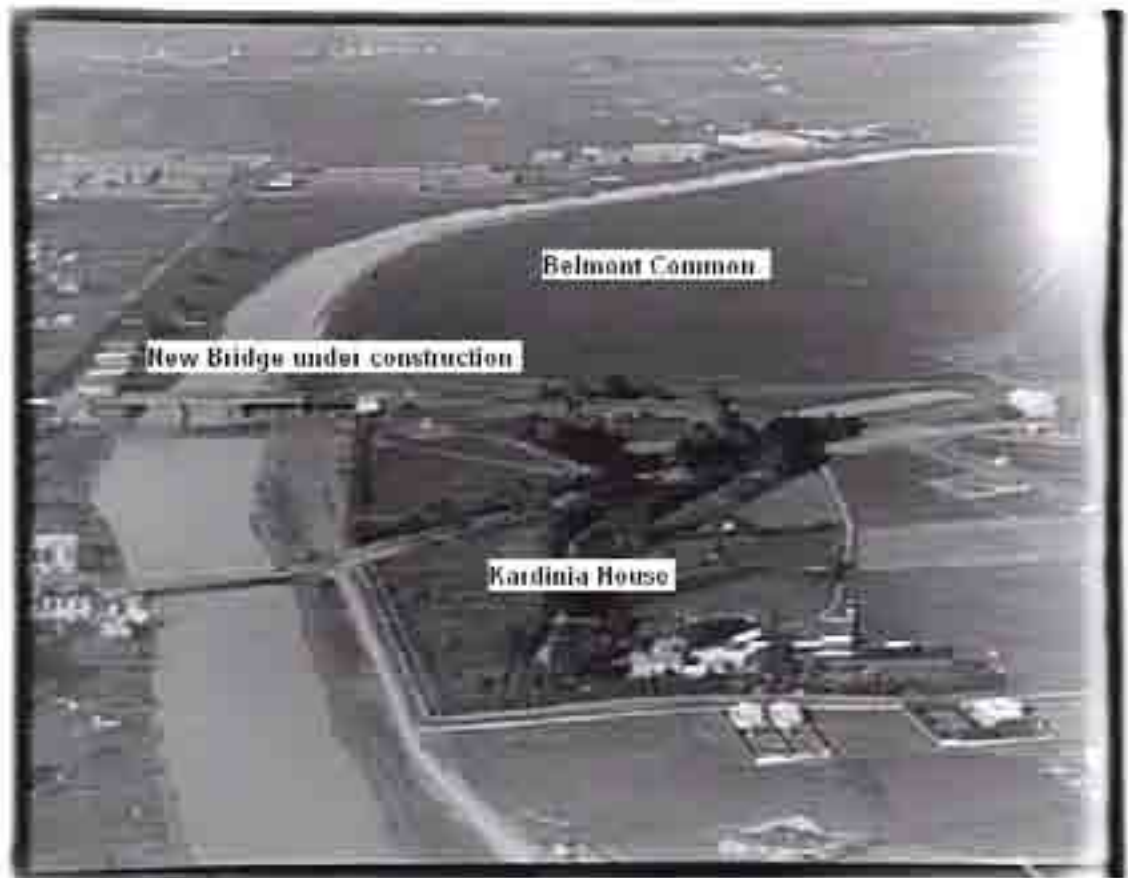
Figure 5.8: Aerial photograph of Belmont, c.1925. showing bridge under construction (middle ground) and Kardinia House (foreground) with tree-lined drive. Note the very few houses constructed fronting Riverview Terrace (foreground). Source: La Trobe Picture Collection, State Library of Victoria, image no. b09211.
