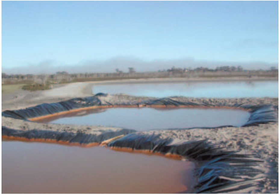
Above: Groundwater flows through two settling ponds to a 90m2 settling basin.
