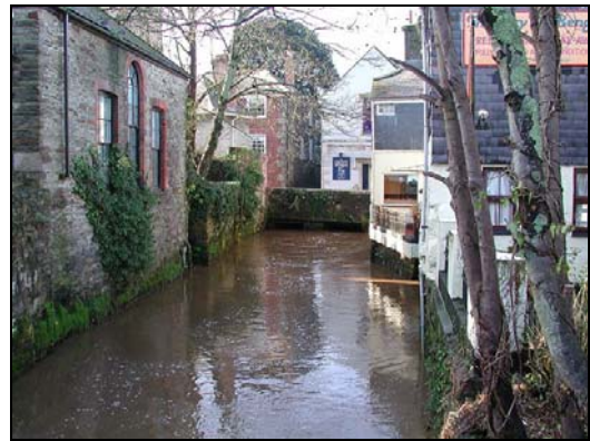
'Old Bridge' on the River Allen. (Photograph: Charles Winpenny, Cornwall CAM.)
