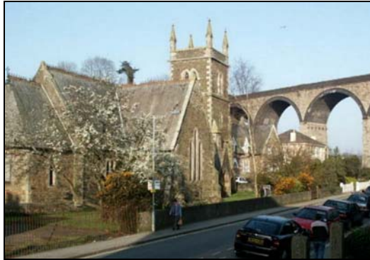
St George's church; the viaduct is a major visual focus in the area.
