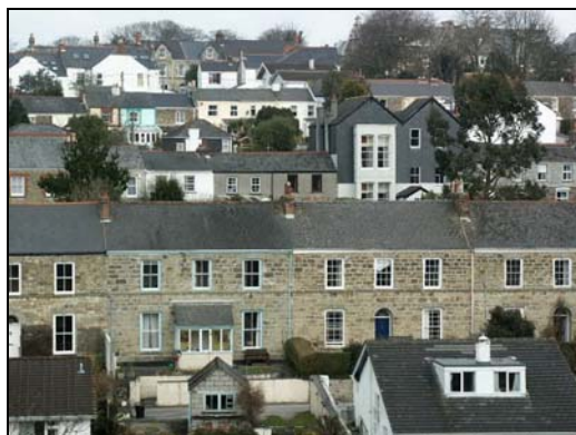
Truro Vean Terrace prominent among the rows and terraces following the contours of the eastern valley side. Trees and greenery are a conspicuous element.
