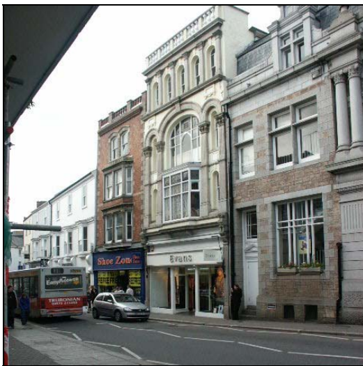
Four-storey elevations on elaborate late 19 th century buildings in St Nicholas Street.
