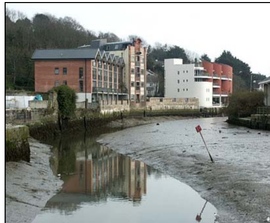
Late 20 th century redevelopment of the historic waterside on the east side of the Truro River. The converted former HTP mill is a prominent feature.
