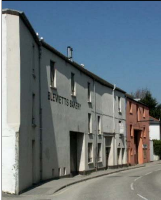
The Malpas Road elevations of historic waterside buildings.
