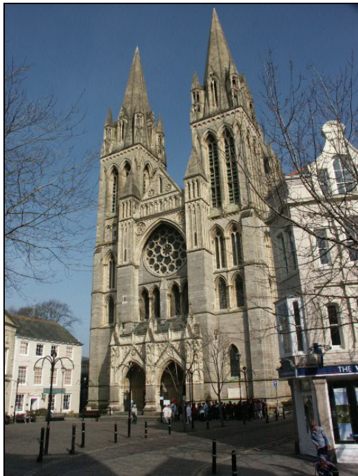
The striking west front of Truro cathedral.
