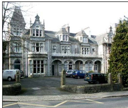
Grandiose design and detail on the late 19 th century Colchester Villas, Falmouth Road.
