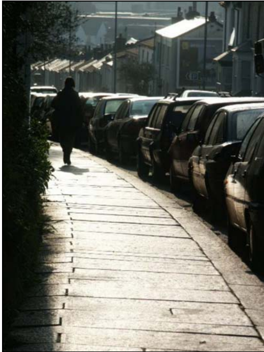
Granite slab surfacing on Richmond Hill.
