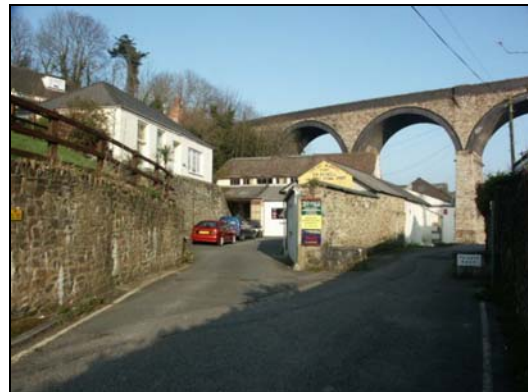
Surviving elements of the Carvedras smelting works, off St George's Road.
