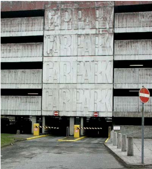
Below: High Cross car park.
