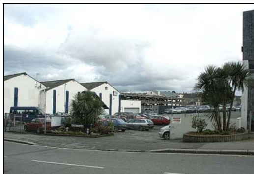
Calenick Street, east side.
