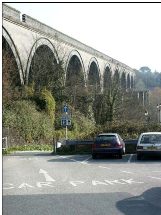
The viaduct creates a strong northern boundary to the area.
