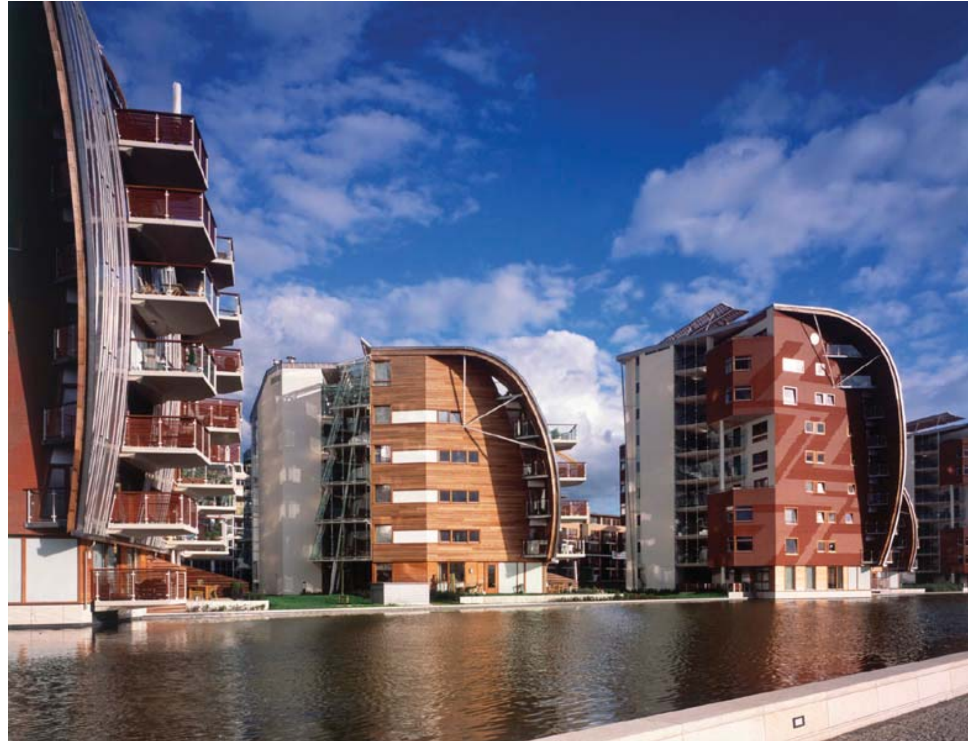
Den Bosch waterside housing, Holland
