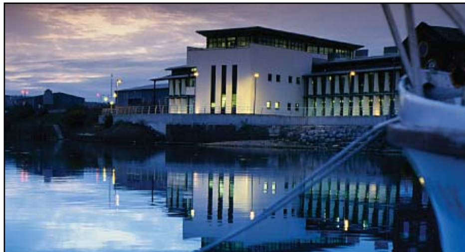
Technium 1 in SA1 Swansea Waterfront
