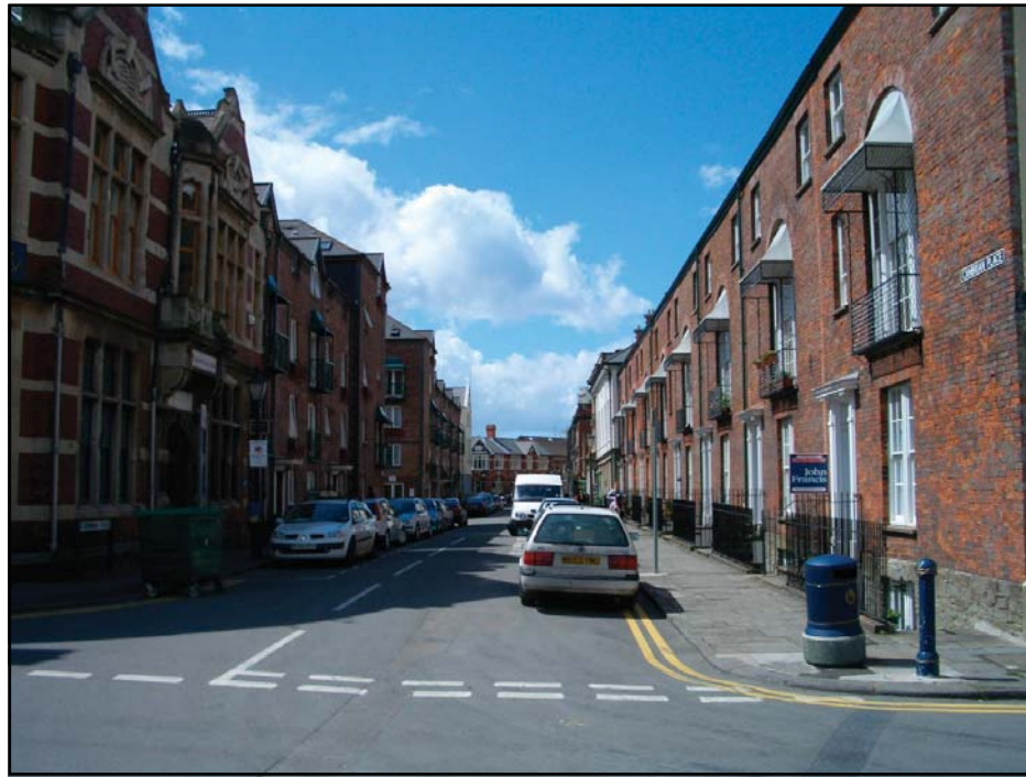
D Maritime Quarter Conservation Area
