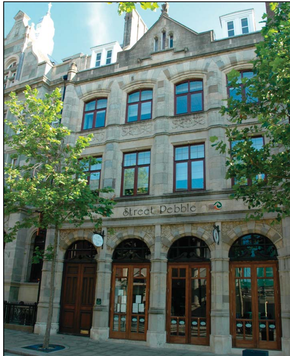
Urban regeneration in Wind Street, Swansea
