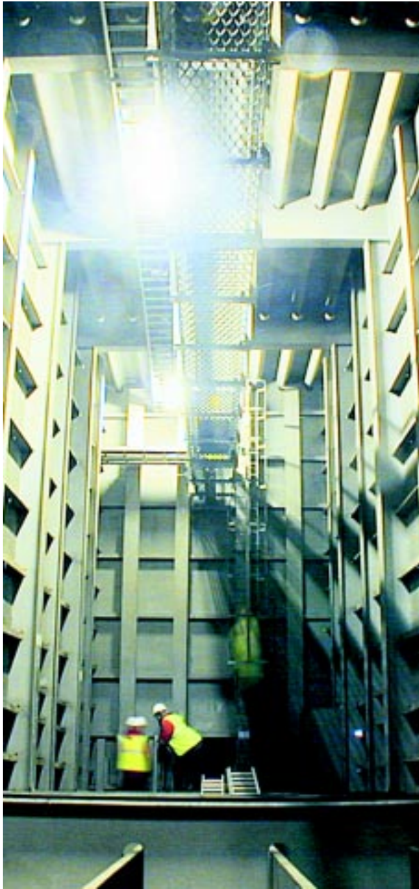
Diaphragm above river pier on Foyle Bridge.
