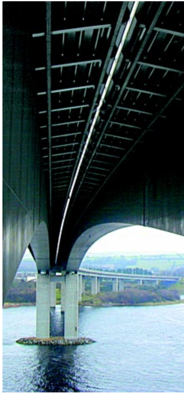
View underneath Foyle Bridge.
