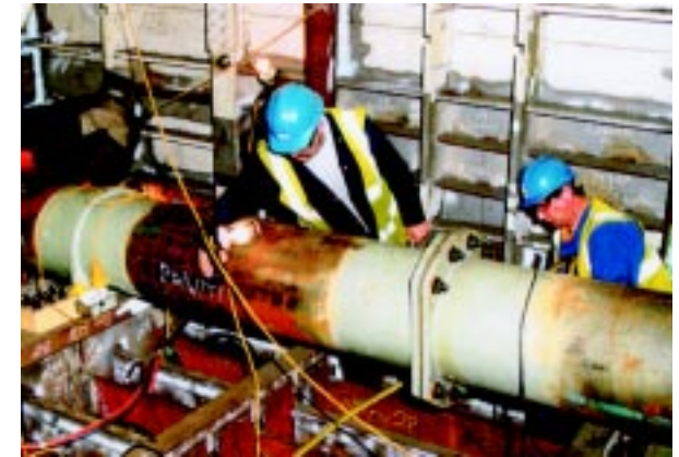
Similar struts installed on another project.
