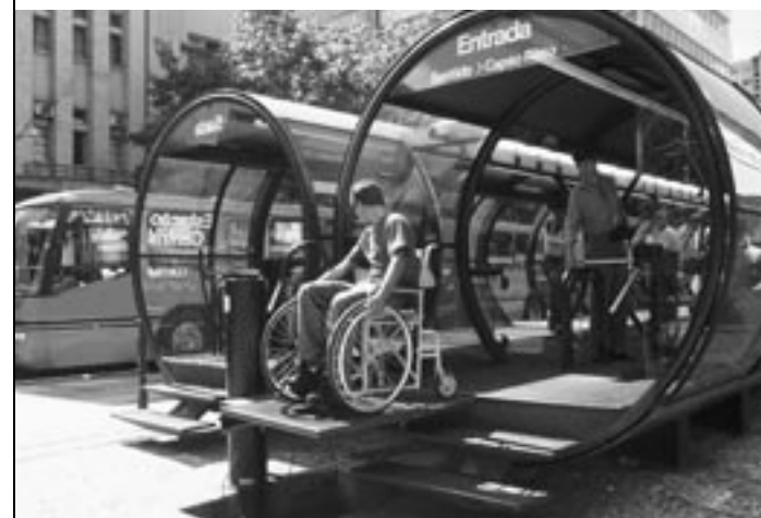
Left View of bus boarding tubes in Curitiba. Fares are paid on entering boarding tubes, which are elevated to bus entry level. Elevator platform raises wheelchair bound riders to door level before bus arrives. Both of these devices speed the transit time for riders.
