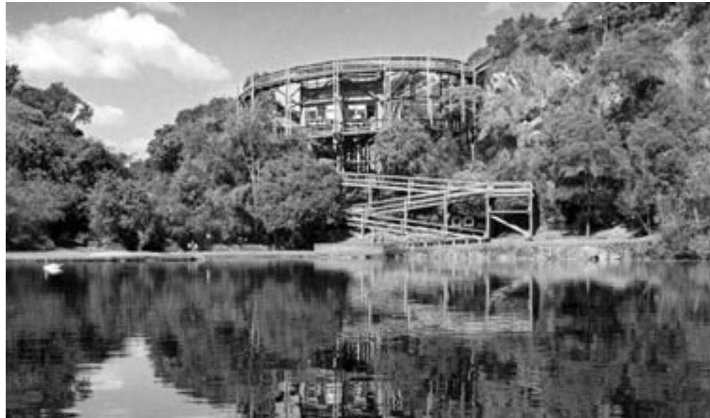
Free University for the Environment, Curitiba, 1992. Designed by Domingos Bongestabs. The building, located in a reused granite quarry, is built from re-claimed eucalyptus wood utility poles.
