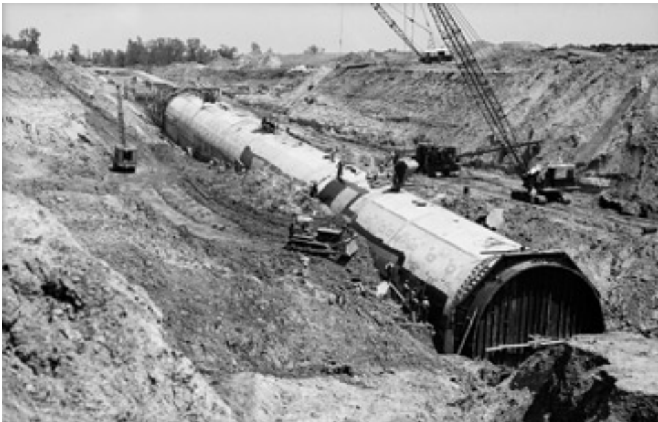
Construction of the approach tunnel. (Photo: TxDOT)
