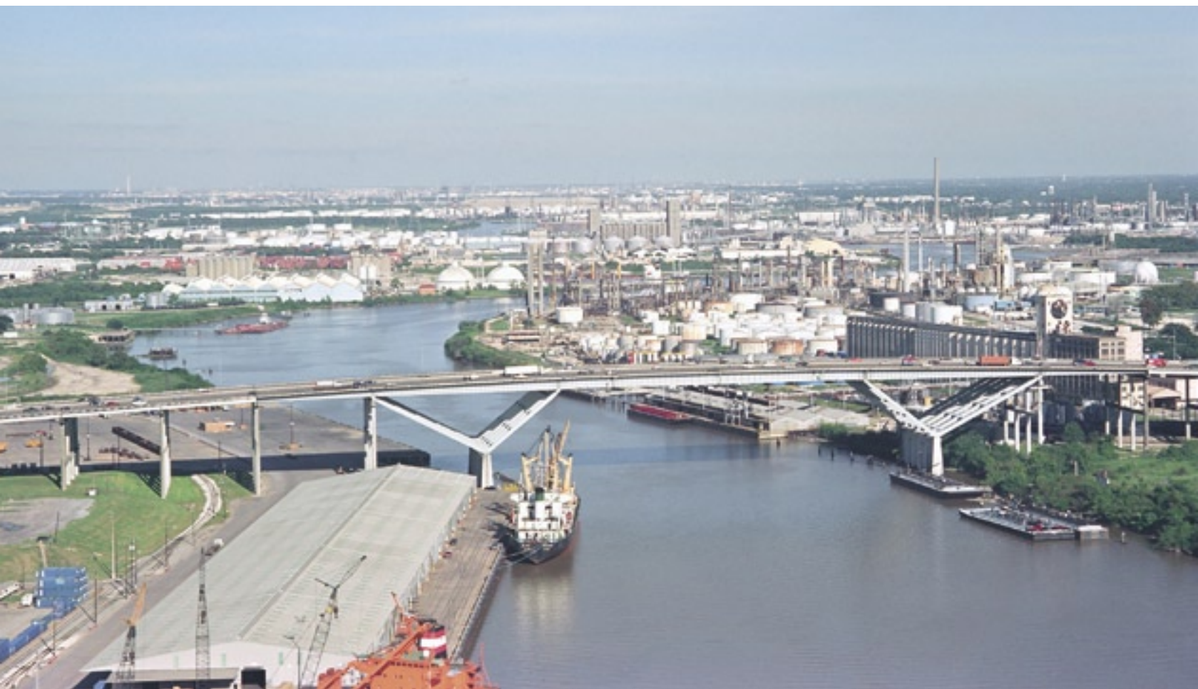
Height is bad: This view looks east along the Houston Ship Channel at the Sidney Sherman Bridge. The 135-foot (41 m) vertical clearance of the bridge caused controversy in the bridge's early years and eventually resulted in collisions with vessels. (Photo: September 2002)
