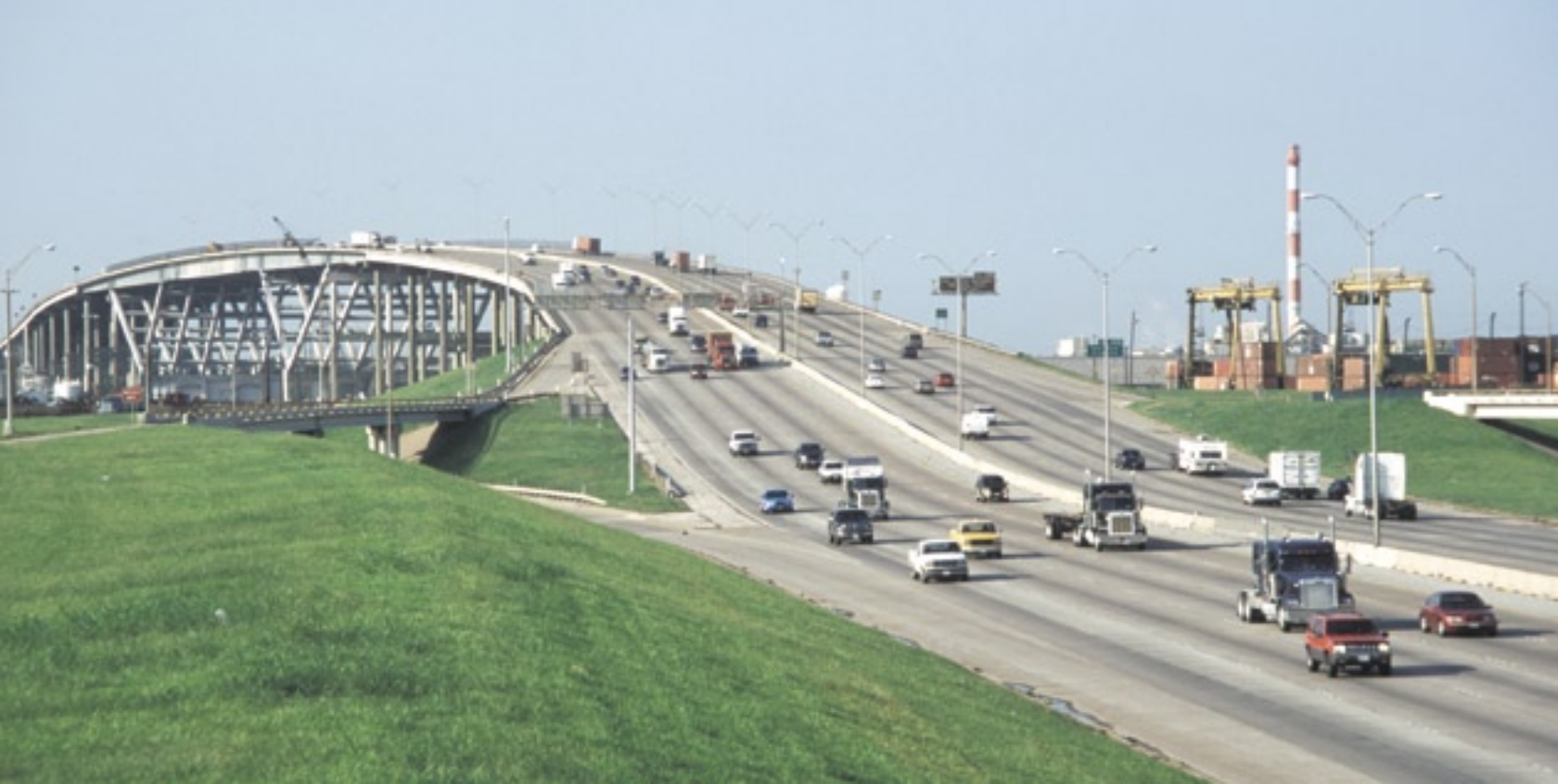
Width is good: The bridge features a deck 152 feet (46 m) wide to accommodate 10 traffic lanes. This view looks south. (Photo: July 2002)
