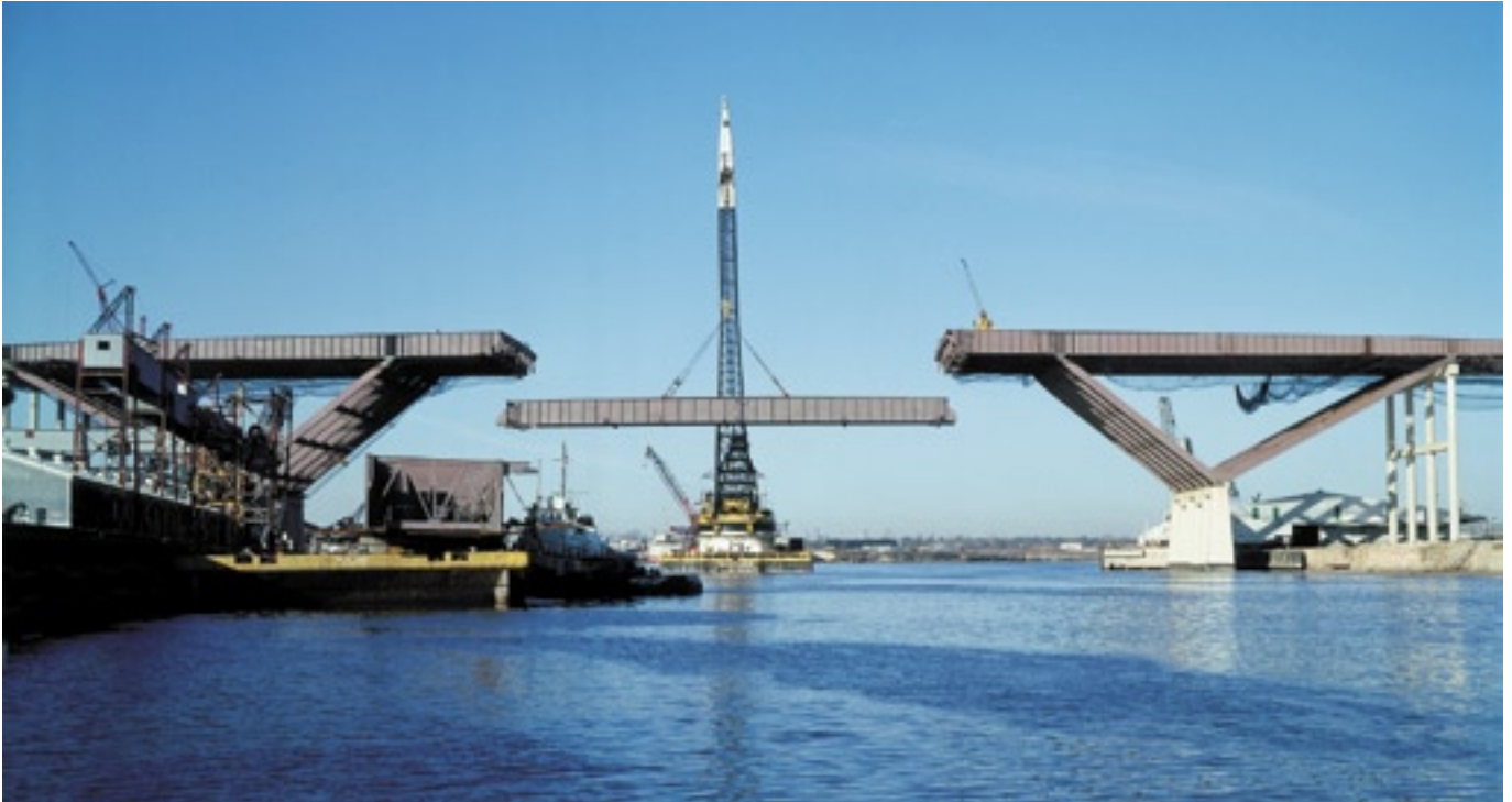
Closing the span: This view shows placement of the first main span girder for the bridge on February 19, 1972. As soon as this beam was in position, the low clearance of the bridge became painfully clear to officials at the Port of Houston. (Photo: TxDOT)
