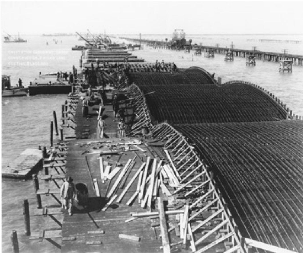
Construction of the first concrete bridge, circa 1911: After the devastating 1900 storm, the need for a bridge capable of surviving hurricanes was clear. Work on a new concrete structure began in 1909 and was completed in 1912. (Photo: Rosenberg Library G-18221FF2, Galveston)
