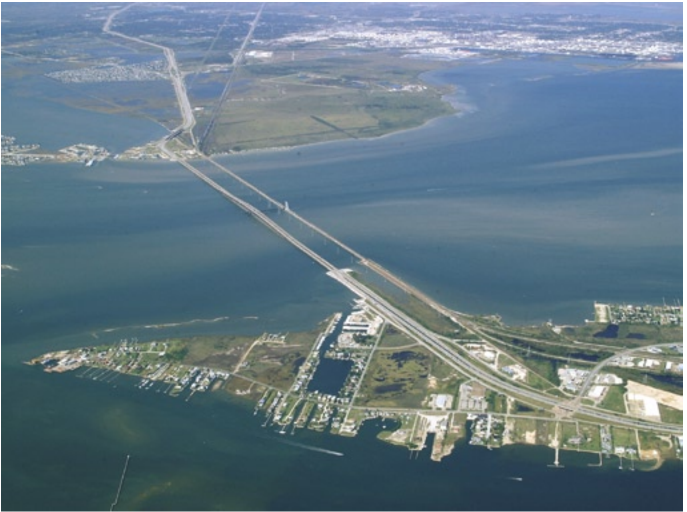
The Galveston Causeway, October 2001: This view looks north, with Galveston Island in the foreground and the mainland in the background. The new causeway structure will be built on the same location as the existing causeway. (Photo: The Positive Image)
