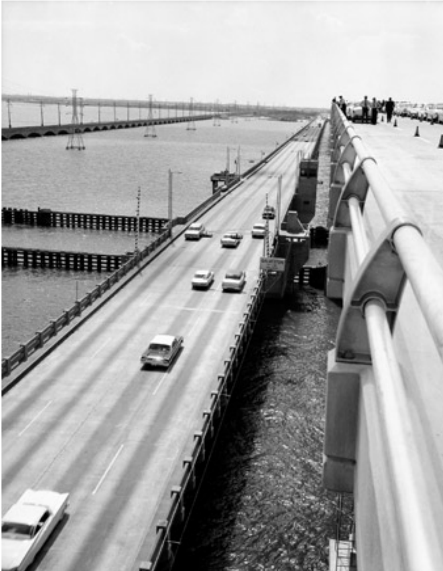
(Left) Dedication of the first high-level span, July 26, 1961: This view looks down on the drawbridge of the 1938 highway structure, which would be replaced by a high-level span in the following years. The first high-level span shown in this photo was constructed with light-weight prefabricated concrete beams which deteriorated more rapidly than expected. By the mid-1970s repairs were required, and by the late 1990s replacement of the bridge became necessary. (Photo: TxDOT)
