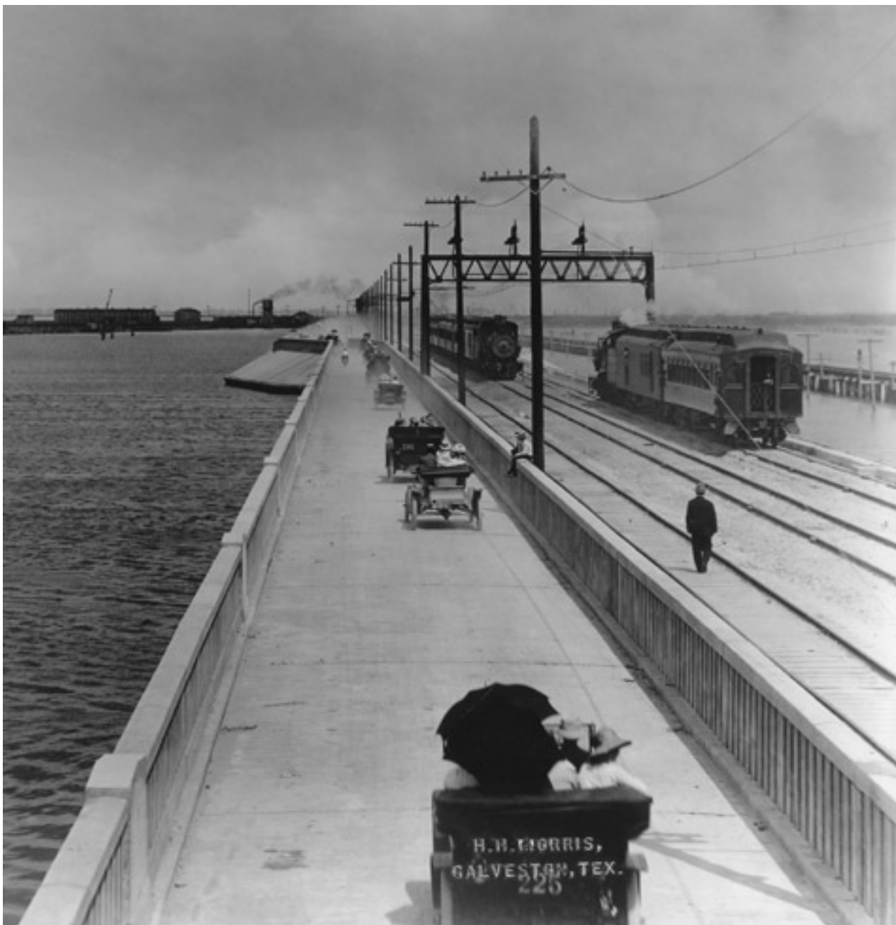
The Galveston Causeway, circa 1912: The first concrete bridge structure was officially dedicated on May 12, 1912. The causeway had two steam railway tracks, one track with overhead electrical wires for the Galveston-Houston Electric Railway, and a vehicular roadway. (Photo: Rosenberg Library G-18221, Galveston)
