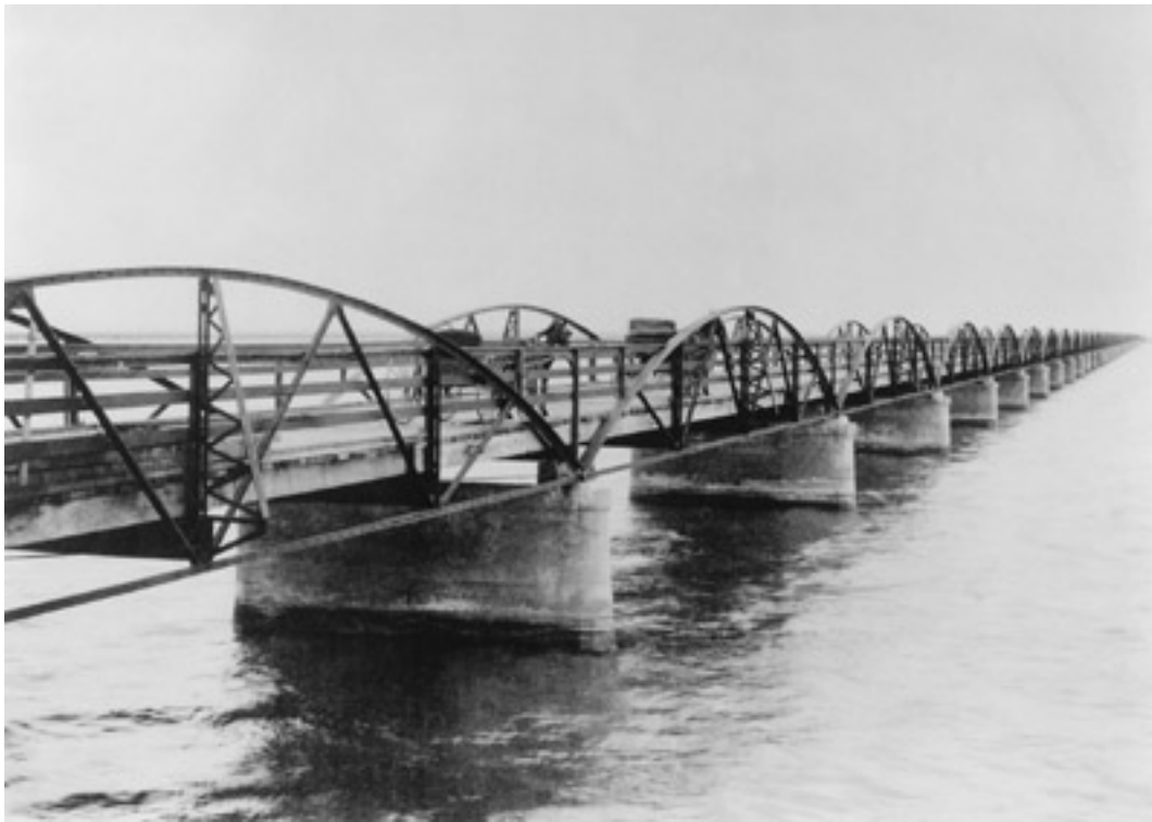
The wagon bridge: The first vehicular crossing of Galveston Bay was the wagon bridge, completed in 1893. The bridge consisted of 80-foot-long (24 m) steel truss spans on concrete piers. This photo shows two horse-drawn carriages on the bridge. The bridge was destroyed in the 1900 hurricane and was not replaced. (Photo: Rosenberg Library, Galveston)
