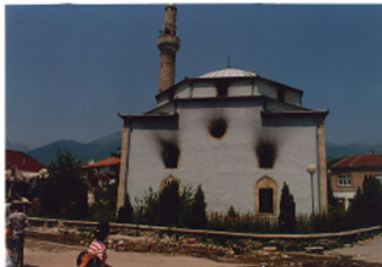
photo by: Xhavit Lakaj (7/99) showing soot marks of fire, intact exterior
