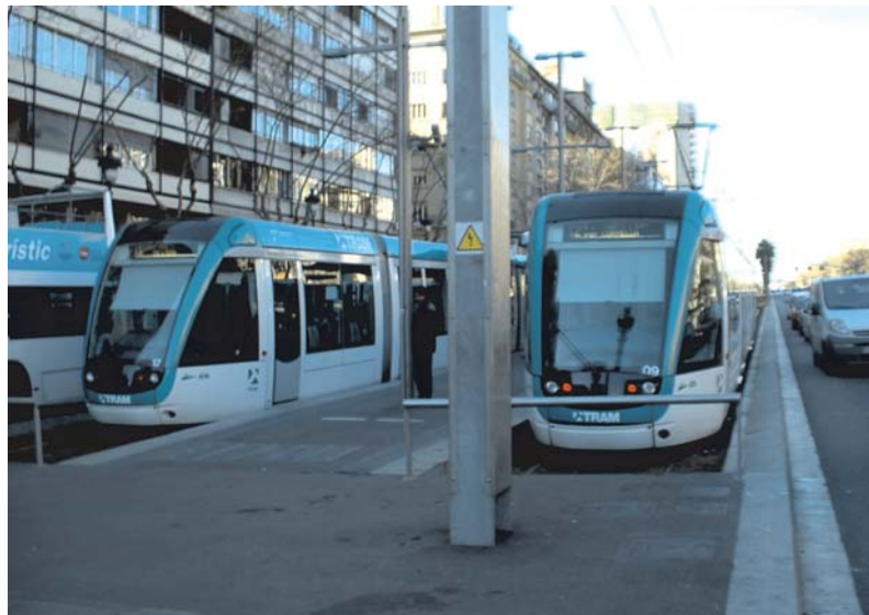
Light metro in Barcelona, Spain
