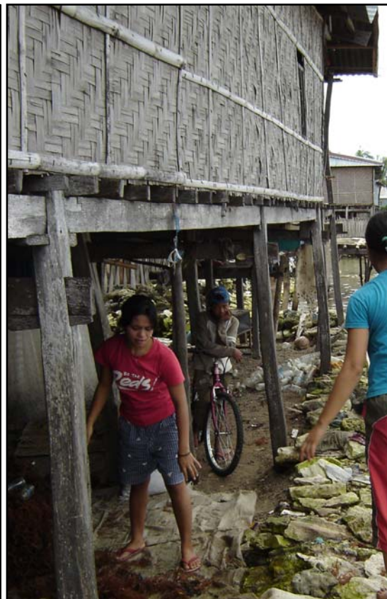
Figure 15. A house on stilts: suitable for mudflats in the intertidal zone.
