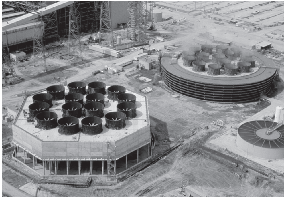
Figure 5—Multifan common plenum cooling towers
