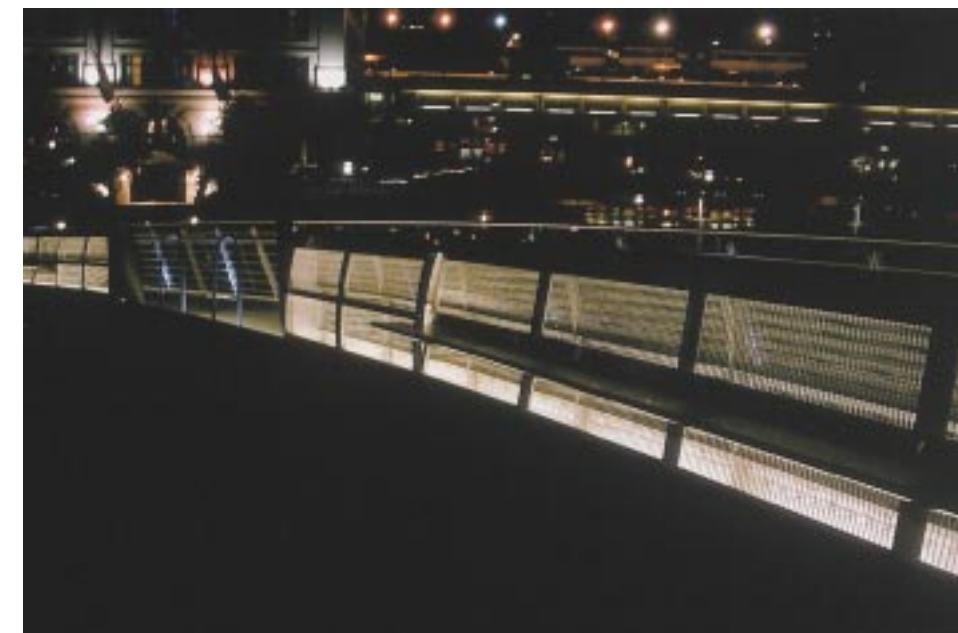
Low energy, long-life LED luminaires delineate the outer edges of the bridge, highlighting the balustrades. The central hedge separating pedestrian and cycle pathways is internally illuminated using low-voltage cold cathode. It also provides low-level lighting across the cycle path deck.
