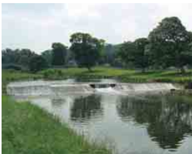
River Bela, weir at Milnthorpe
