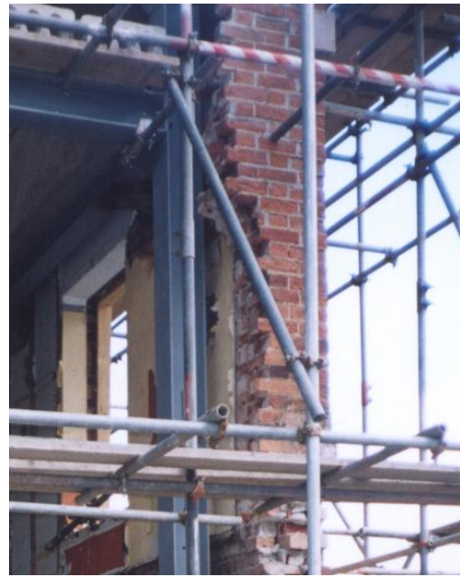
Photograph 2 (note the lack of insulation improvement to the retained facade)
