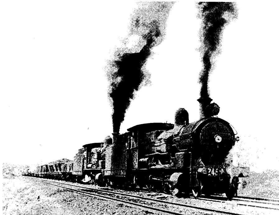
Coal and freight trains were hauled, until dieselisation, mainly by "standard goods" type locomotives. In the twilight years of steam, a "double-header" struggles out of Waterfall yard, bound for Enfield, 26/9/1964.
